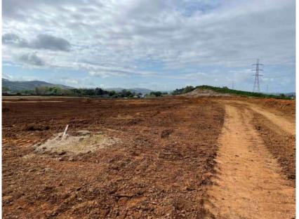
**Looking north west** – View from ridgeline. Material comprising clayey silt with basalt gravel inclusions. At time of photo taken, ridgeline has been cut down by 1 m.
