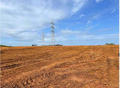
**Looking east** – Cut sequence into ridgeline which forms the edge of A4. It is expected that a further 3 meters of cut required to achieve design levels.
