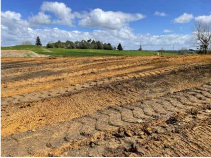
**Looking east** - AVF silt exposed following topsoil stripping works.
