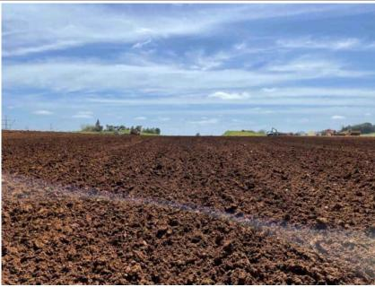
**Looking south** - Season 1 filling at A11 being disked and allowed to dry prior to recompacting and recommencing filling.
