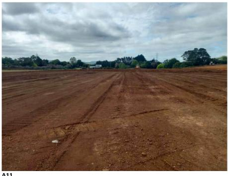
**A11**Soil is trimmed and drying before recompacting.
