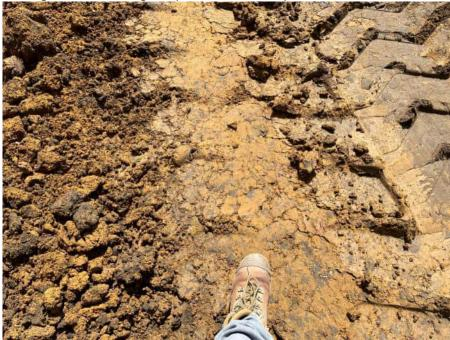
Exposed subgrade comprising, AVF clay & silt. Some topsoil stuck in wheels have been left behind by motor scraper.
