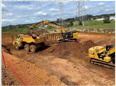
Looking north east – northern edge of pond being excavated. Cut material taken to stock pile for blending.
