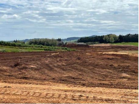
Looking west – Cut material having been disked and let to dry prior to being removed and placed at stockpile at A6/A7.
