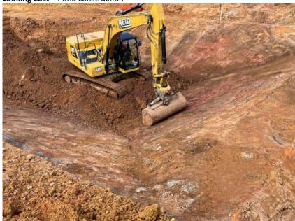
Construction of sediment pond side walls does not appear to show instability at 2v:1h. Material consists of predominantly clay & silt with highly to completely weathered basalt. The variability in soil type apparent in the sediment pond construction is consistent with weathered basalt flow features.
