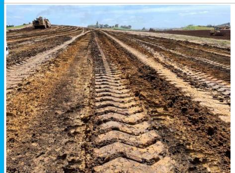
Looking north - Trimming of topsoil material to exposed volcanic soils.
