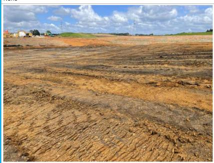
**Looking north east** - Extent of topsoil stripping exposing subgrade.
