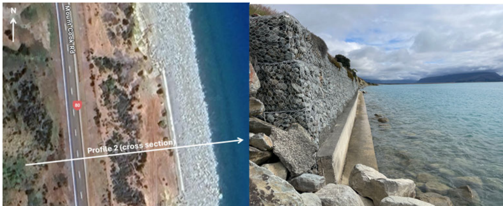
Figure 9, riprap protection is provided for the toe of the wall however the vertical/lateral extent of the protection is unknown.
