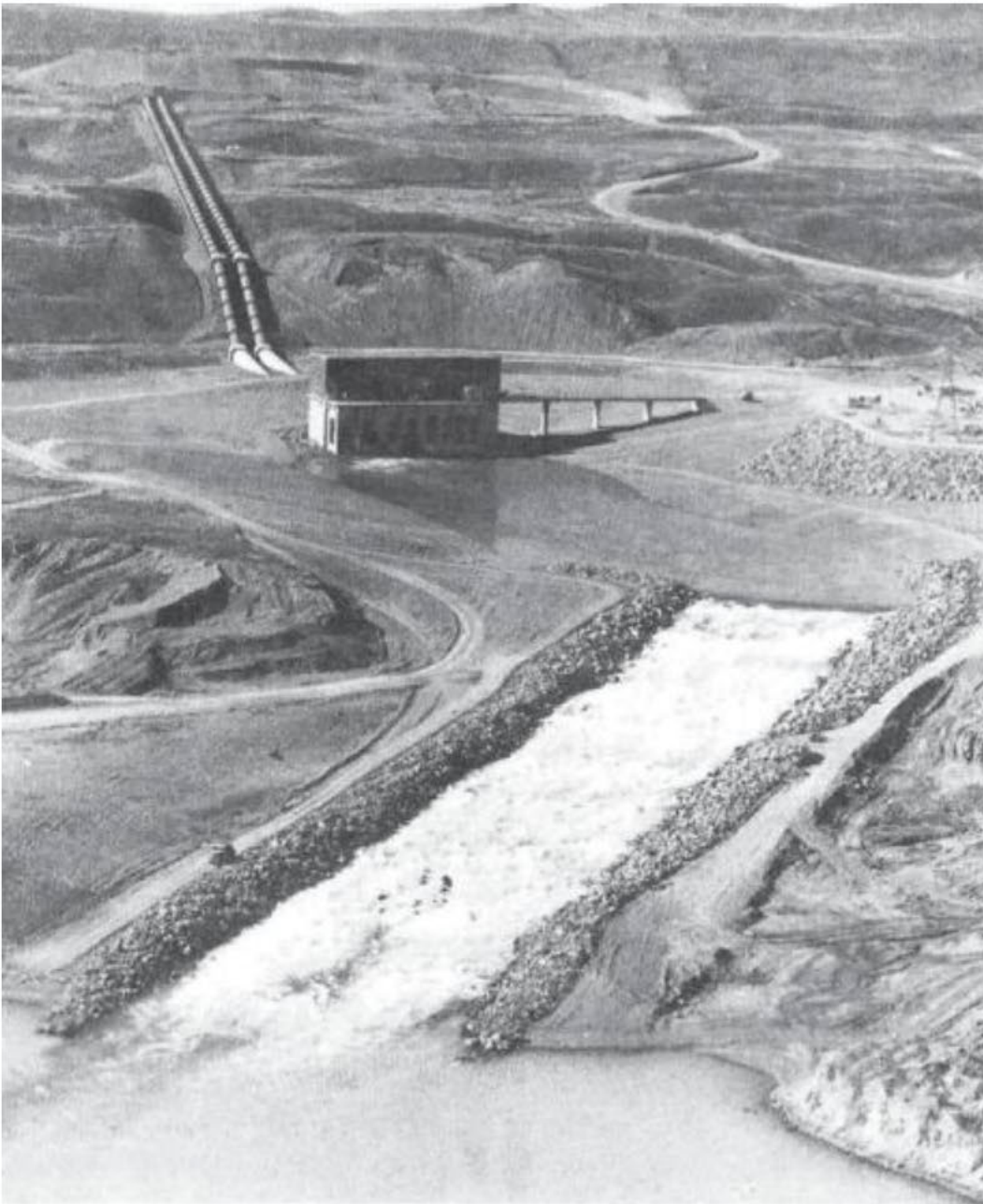
Figure 2.1: Oblique aerial view of Tekapo B Power Station temporary tailrace channel in operation discharging 100 m 3 /s into Lake Pūkaki (date and time of photograph unknown but lake level inferred from as-built drawings to be below level of sill 11 at RL 502.23 m)
