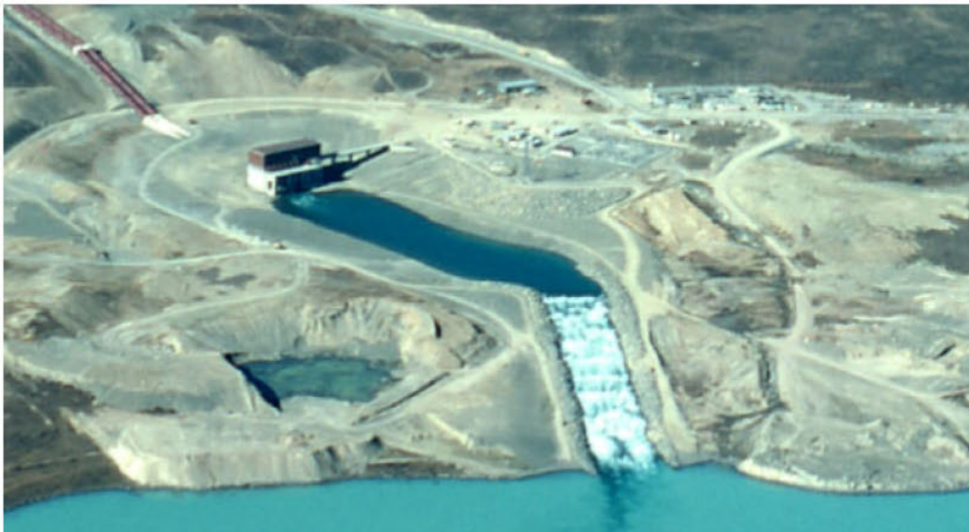
Figure 6 Lake Pūkaki at 504.3 m RL showing the full extent of the tailrace and weir.
