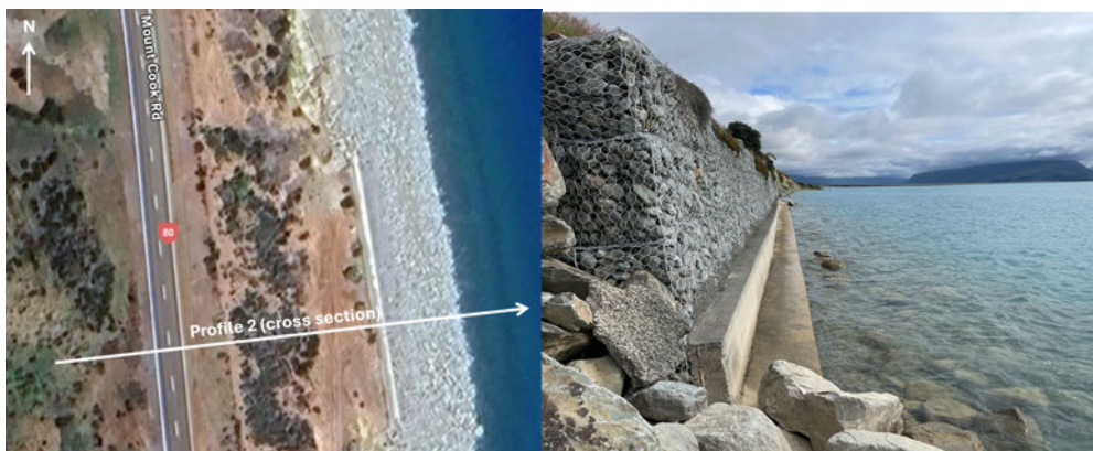
Figure 9 Left: Aerial image of the Gabion retaining wall between SH 80 RS 17 RP 12.64 – 12.7 (Source: Google Maps). Right: Photo taken of the gabion retaining wall facing north.
