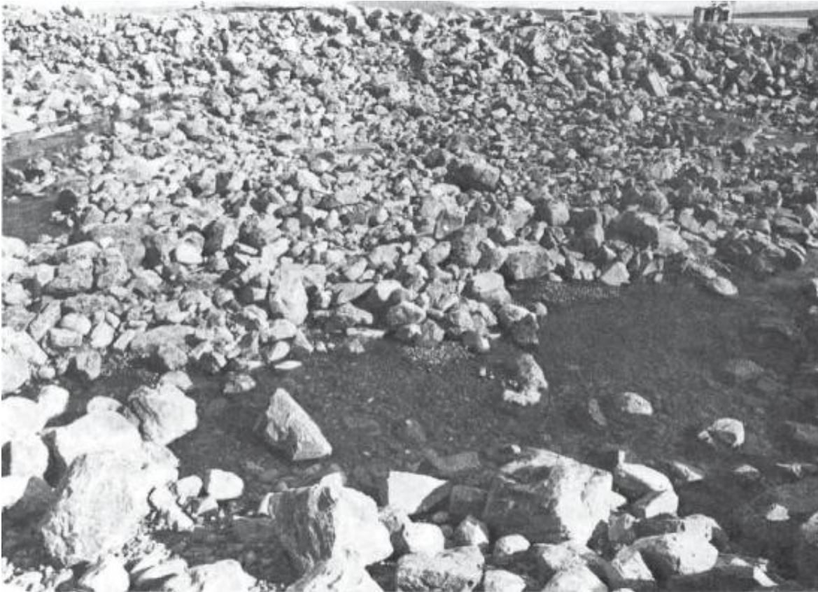
Figure 3.5: View of rock-lined bed between concrete sills 4 and 5 on the chute component of the Tekapo B Power Station temporary tailrace channel
