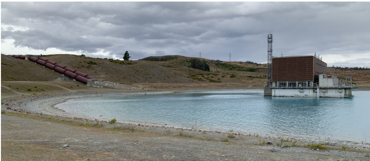
Figure 4 Site visit photo of Tekapo B Power Station showing the two penstocks.
