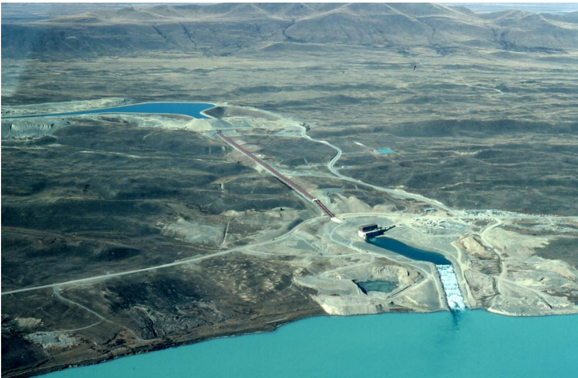
Figure 1.1: Tekapo B Power Station and Canal with temporary tailrace weir and rock chute in operation at bottom right corner of photograph (August 1977)
