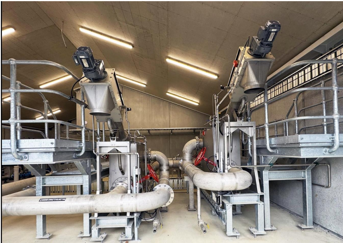
Figure 11 - Fine and Coarse Inlet Screens at a treatment plant designed and built by Apex Water
