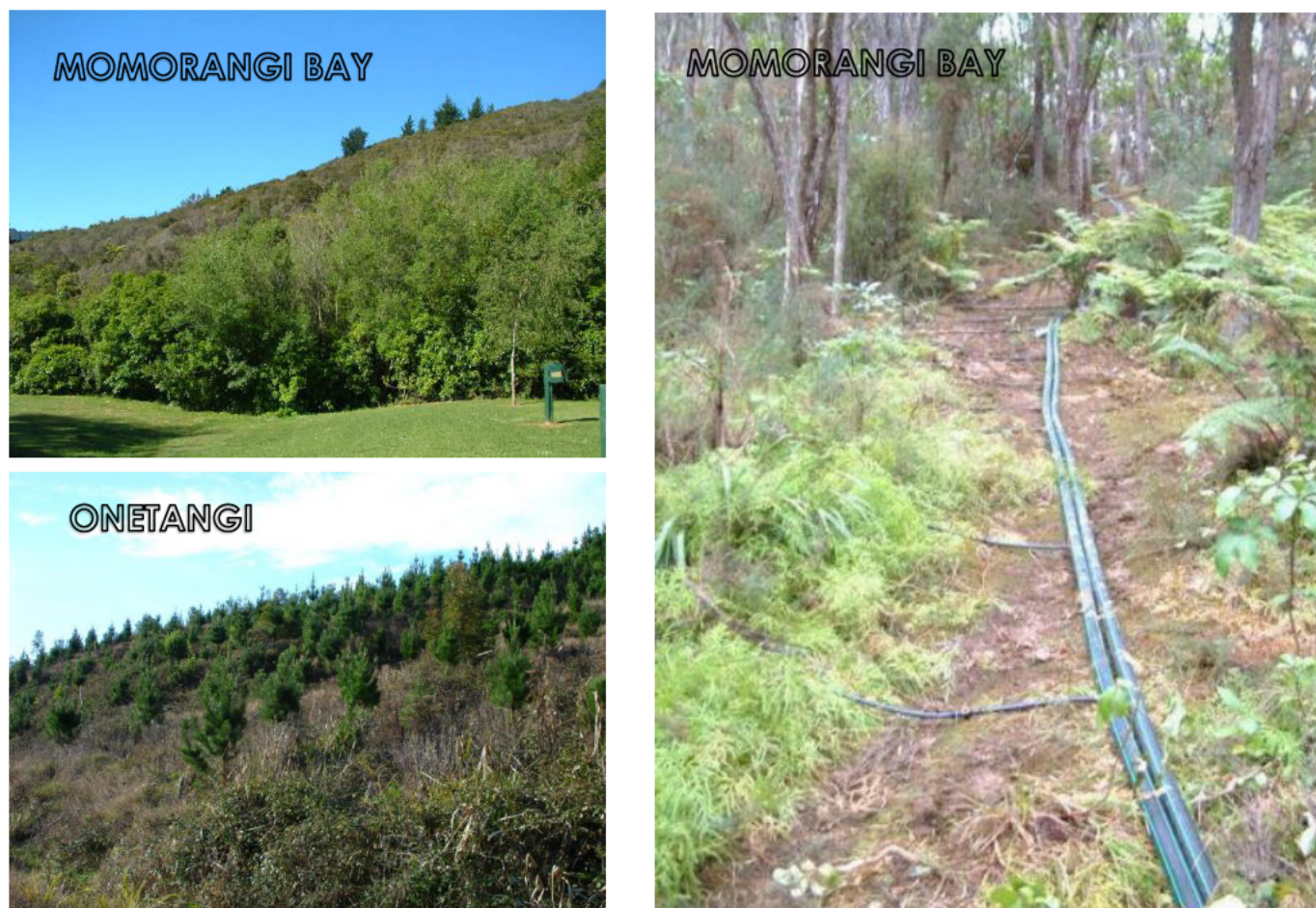
Figure 22 – Examples of surface laid drip irrigation line installation for wastewater treatment plants of similar size and capacity as that proposed.
