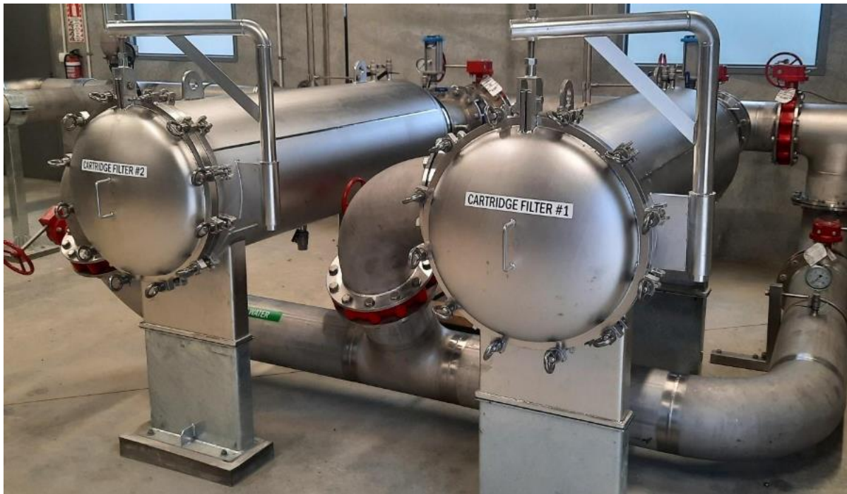
Figure 42: Duty / standby cartridge filter units (Motueka WTP)
