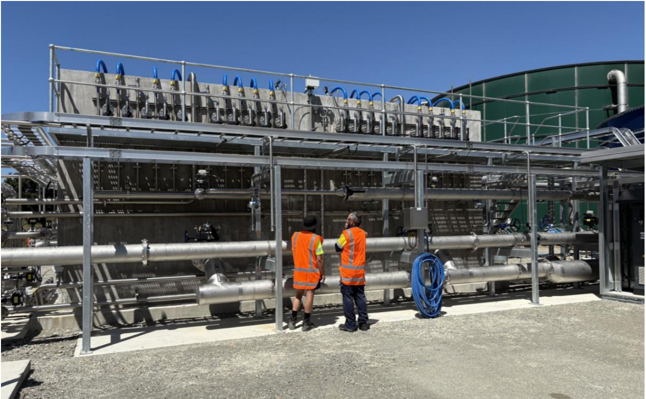
Figure 7 - An MBR Membrane Tank on an Apex Water designed and built dairy site
