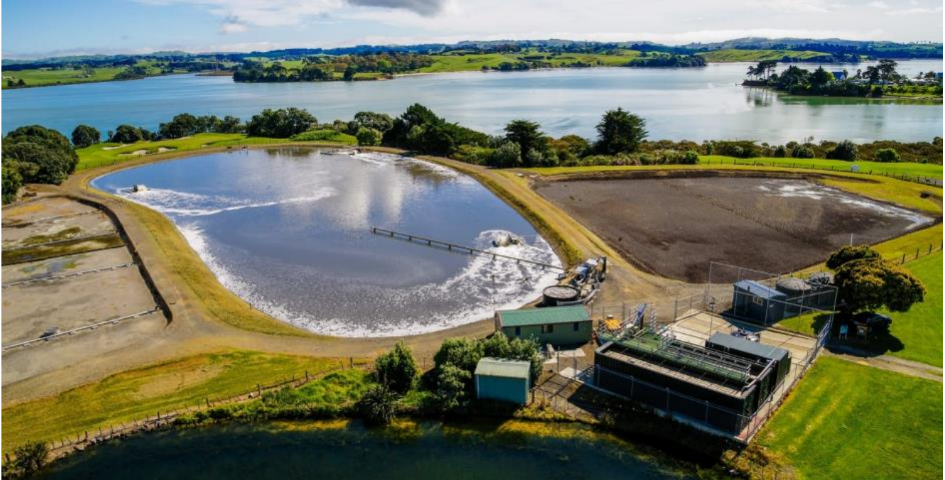
Figure 136 - A modular and containerised MBR treatment plant designed and built by Apex Water for Watercare
