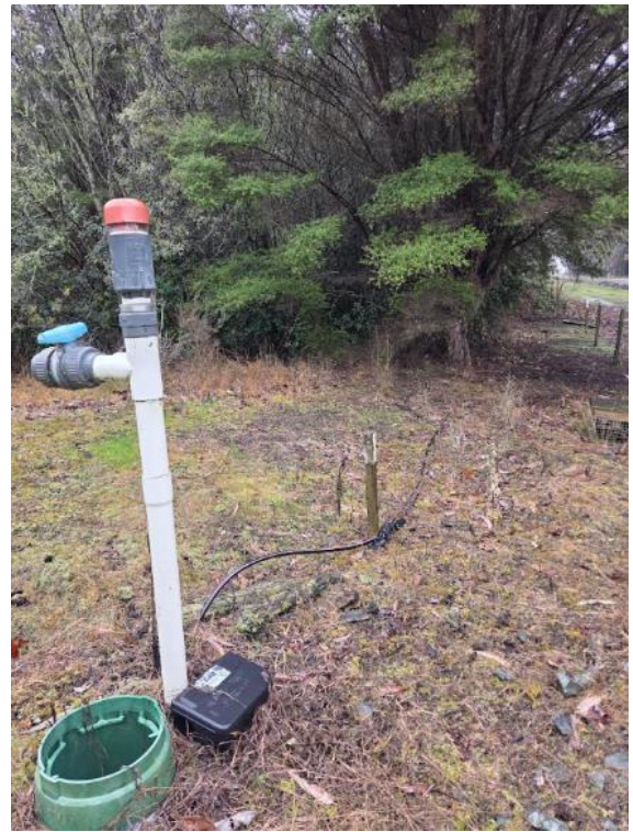
Figure 23 - Omaha Wastewater treatment plant wastewater discharge via surface mounted drip irrigation through both bushy and wooded areas.
