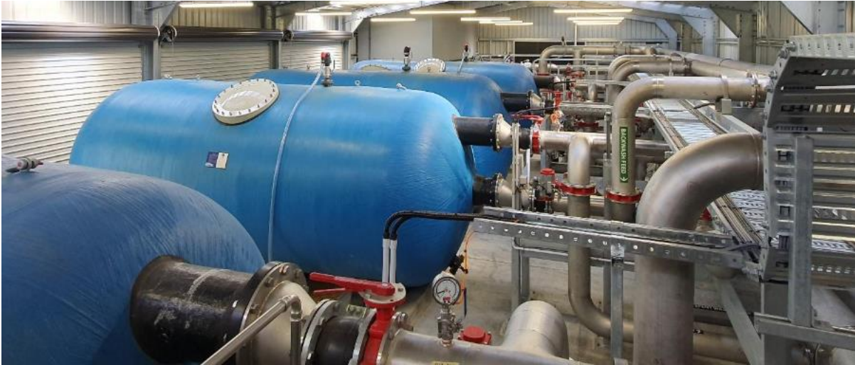
Figure 43: Horizontal multi-media filters (Braemar Springs WTP)
