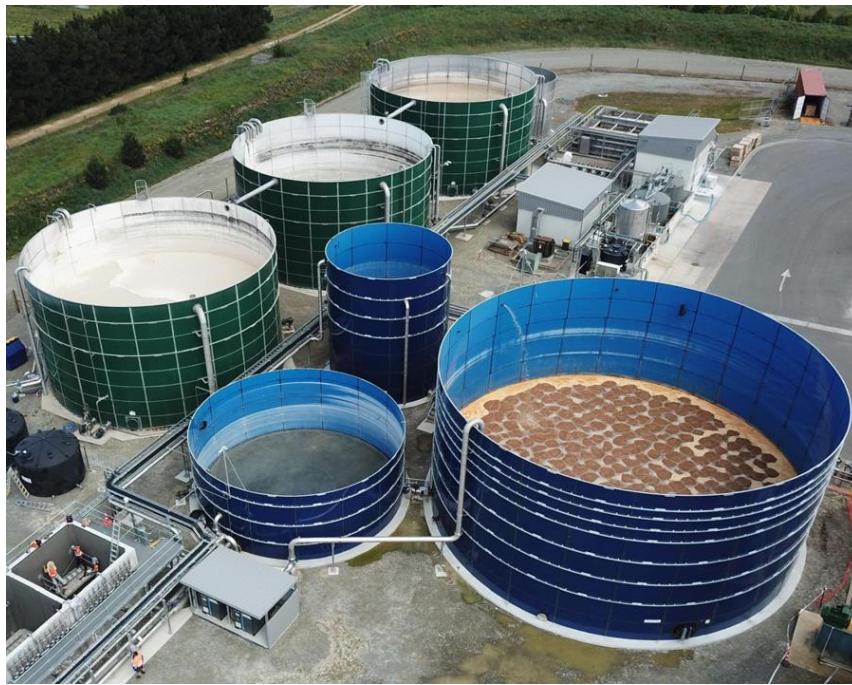
Figure 12 - An Aeration Tank in Action (Large Blue Tank)
