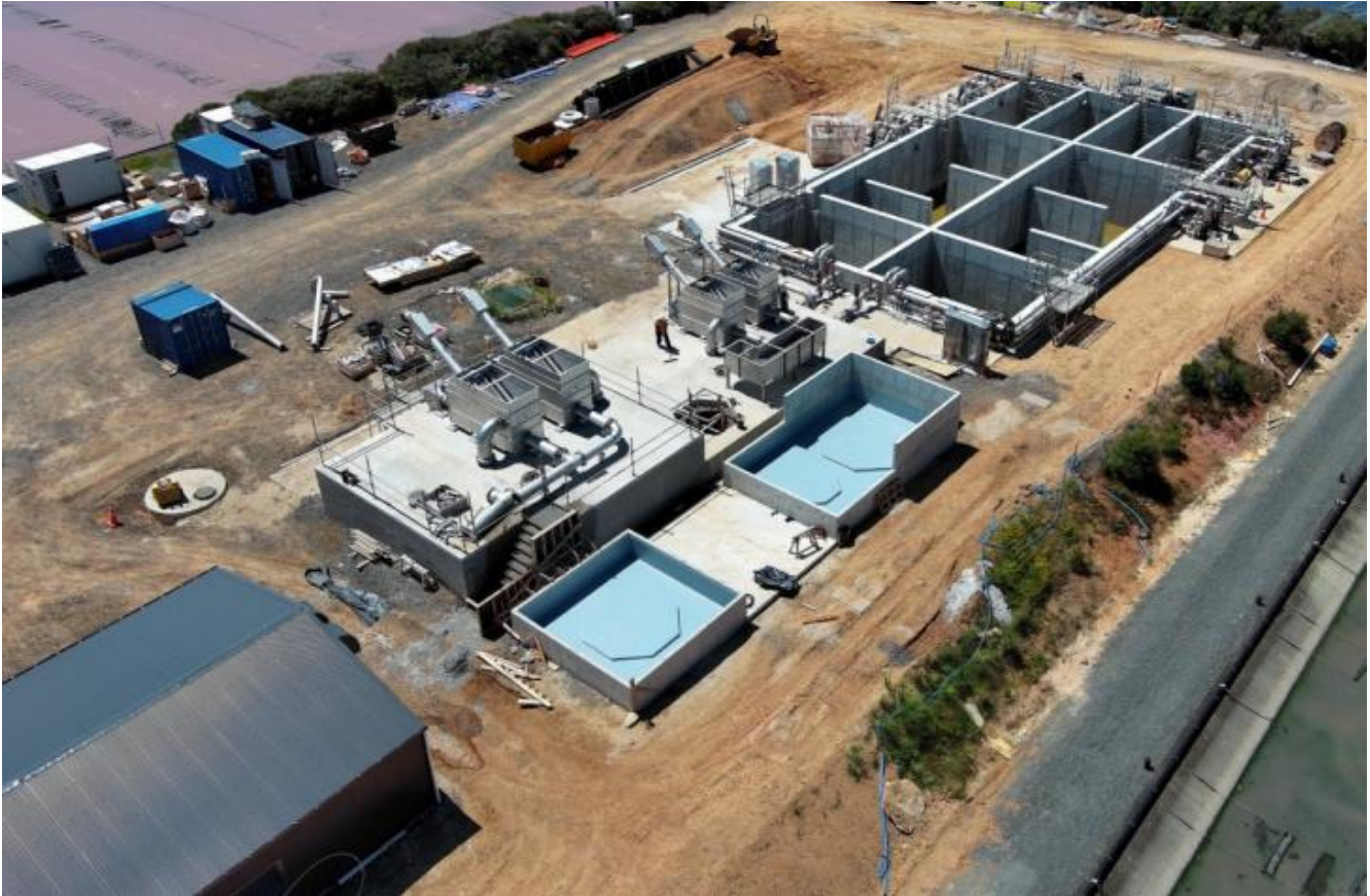
Figure 8 - An under construction MABR/MBR hybrid treatment plant designed and under construction by Apex Water for Watercare
