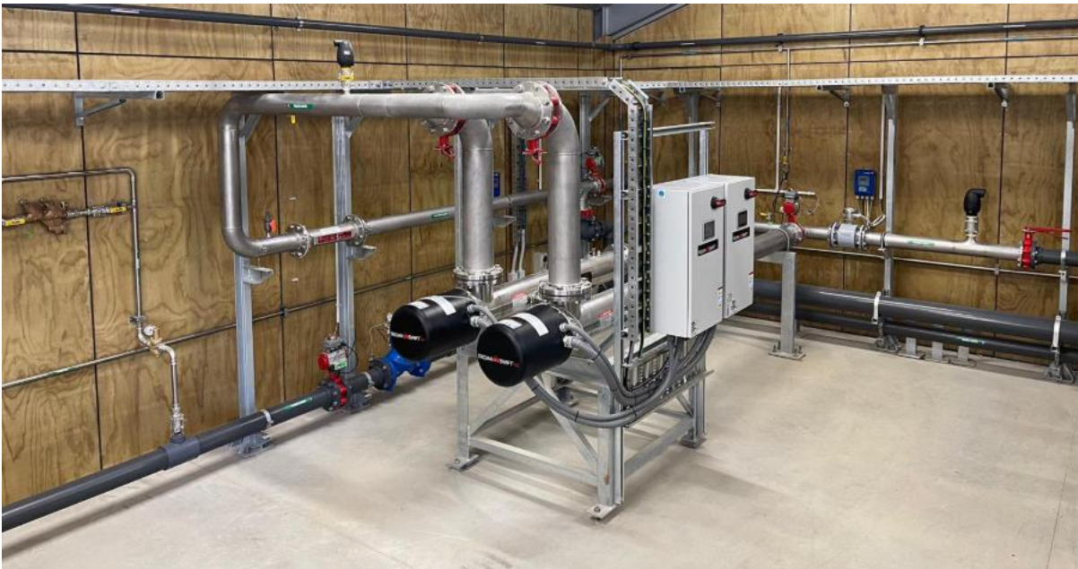
Figure 45: Duty / standby UV disinfection units (Karaka Village North WTP)
