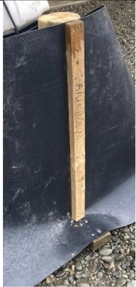
Photograph Appendix H.4: HDPE membrane attached to post.
