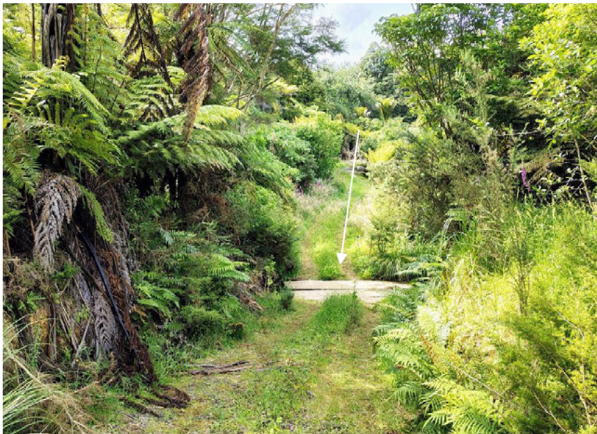
Figure 28. Photograph 4 looking south with a concrete bridge indicated by arrow
