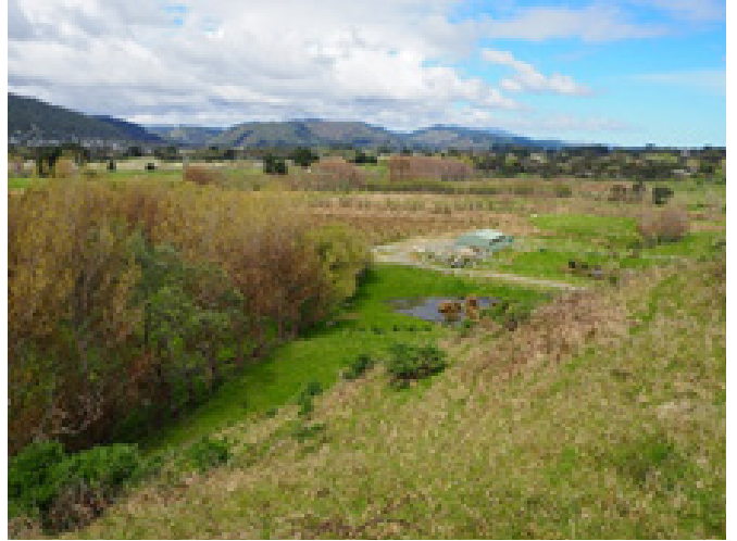
Figure 46. View over part of the central open space and flood retention area
