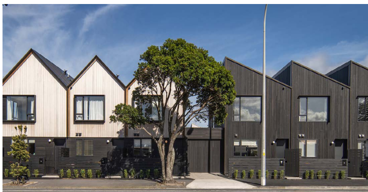
Figure 93. Terrace Housing Hobsonville, Auckland
