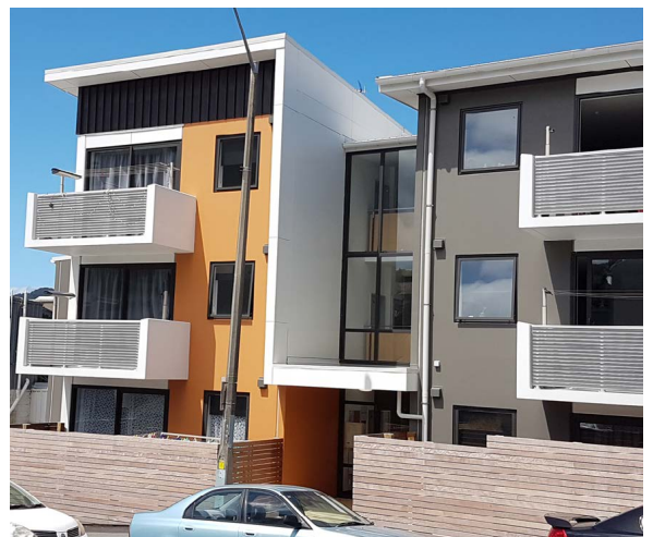
Figure 99. WCC Te Mara Apartments Novak & Middleton, Mount Cook, Wellington
