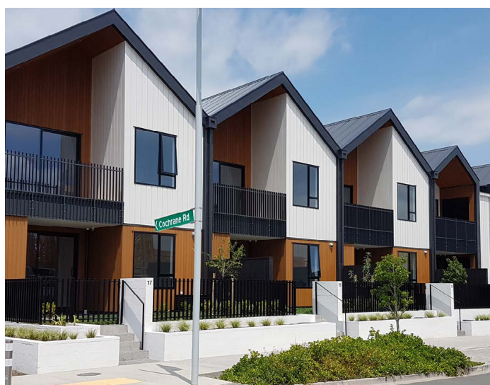
Figure 88. Terrace Housing Hobsonville, Auckland
