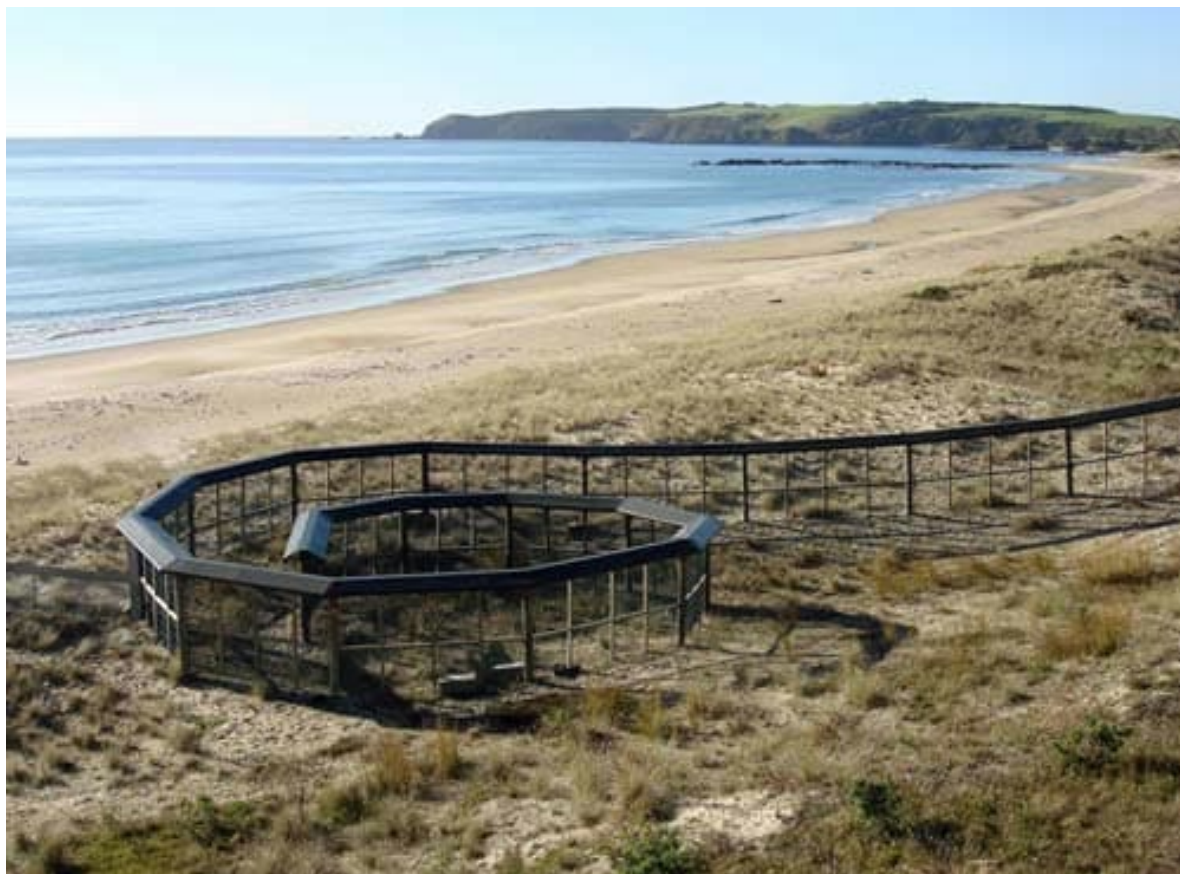
Plate 3. Indicative design of predator exclusion fence with top cap, and end spiral to reduce incursions around fence edges. (photo shows Tawharanui Sanctuary fence).
