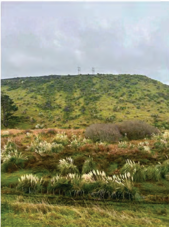
Photo 15: 2nd June- Hill remaining above tributary of Mitiwai Stream and wetland area. Visible sand migration down ridgeline.
