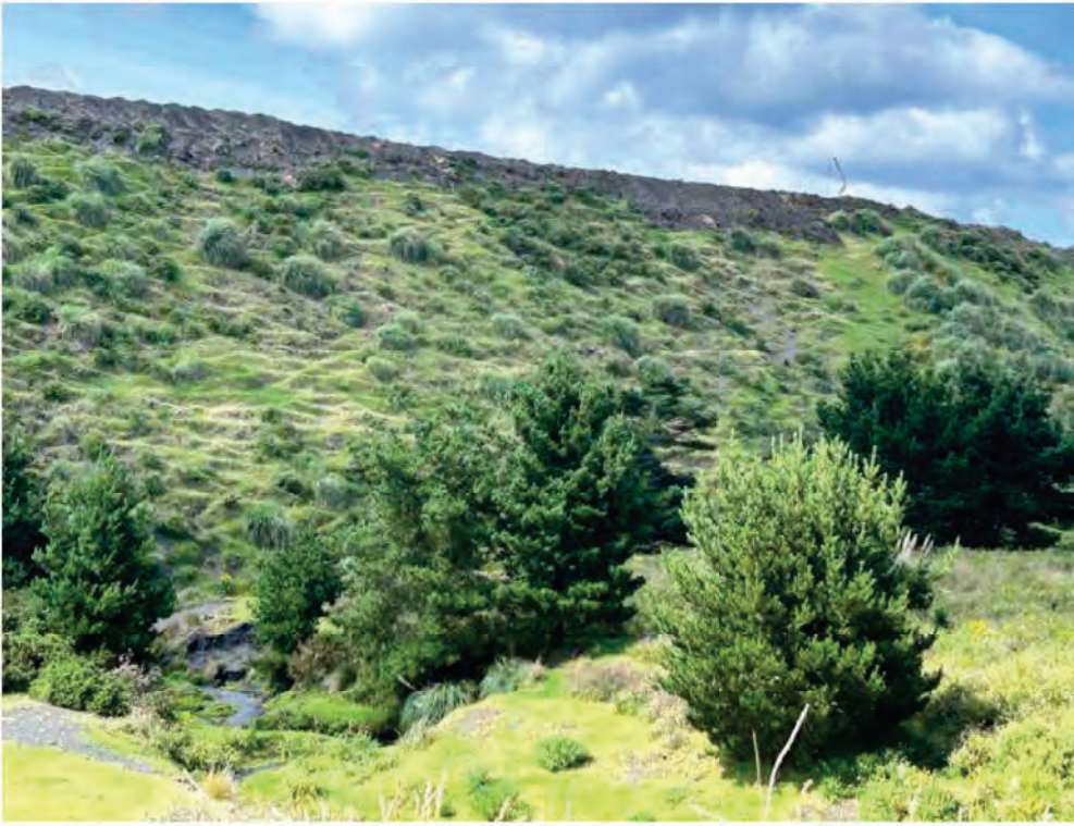
Photo 18: 28 th December 2023- Works above the Mitiwai Stream- westernmost boundary of Wetini land
