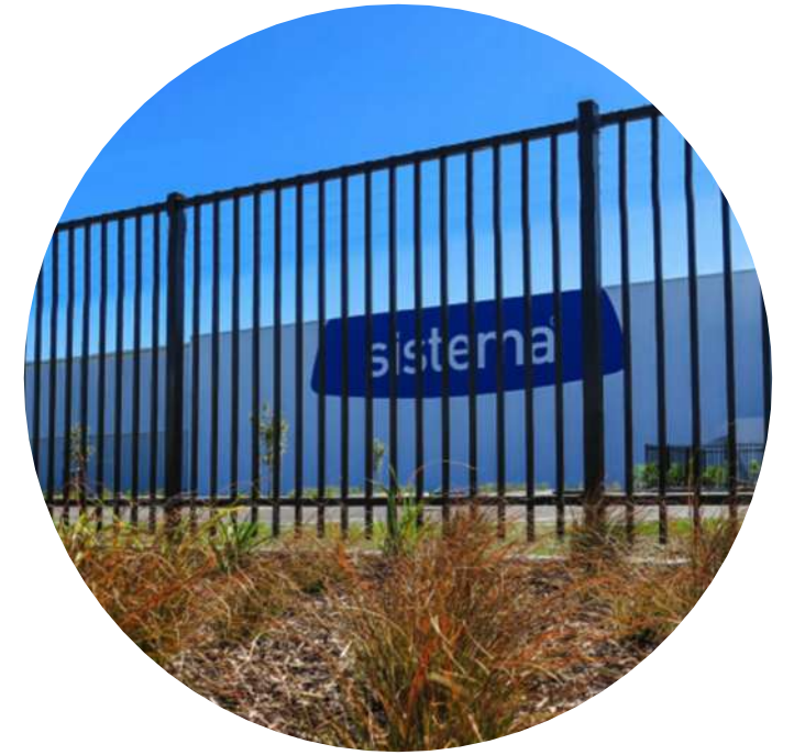
1.8m high open aluminium fence
