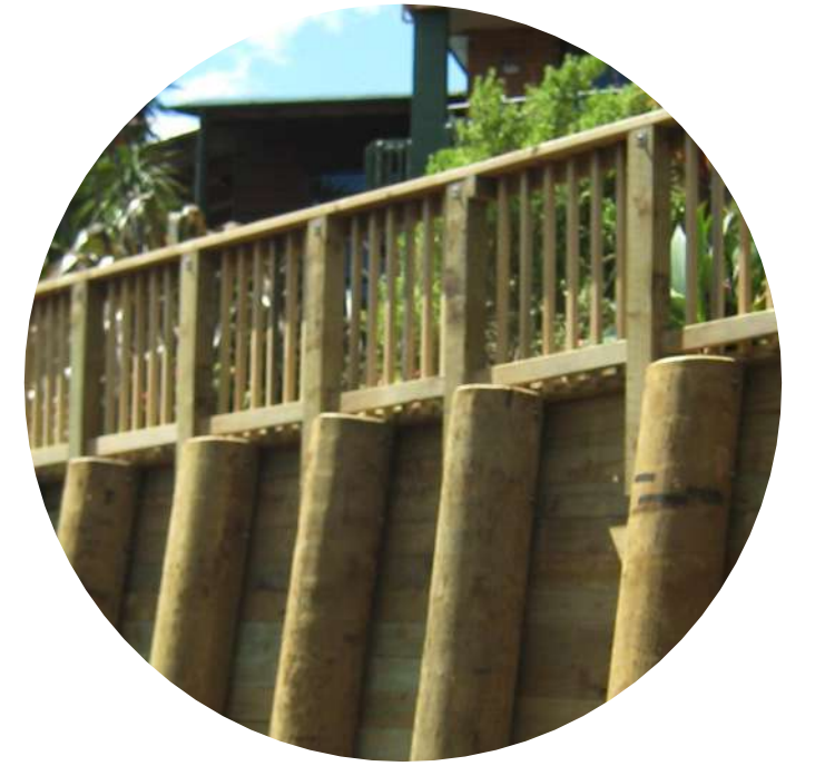
1.1m high timber batten balustrade, within private lots only, staining optional
