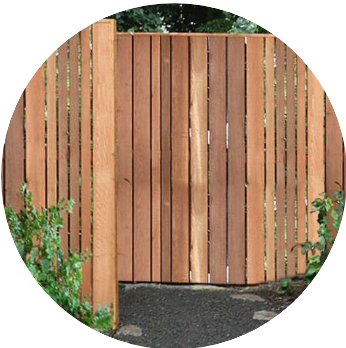
1.5m high varied verticalslatted timber fence, stain / paint finish
