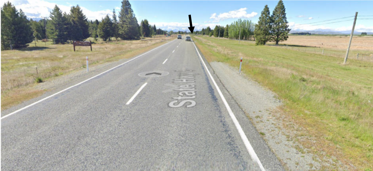
Figure 5.3: Northbound approach (Arrow indicates approximate limit line location in the throat of the accessway) (Source: Google Streetview 2024)
