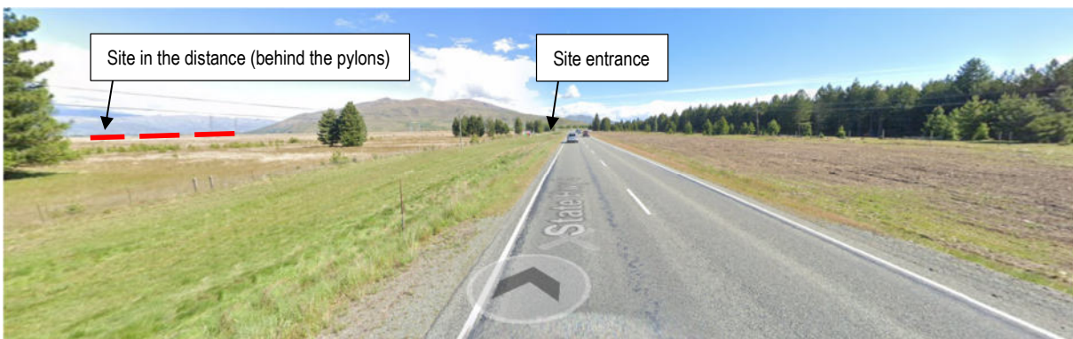
Figure 5.7: Complete view – Southbound approaching site (Source: Google Streetview 2024)
