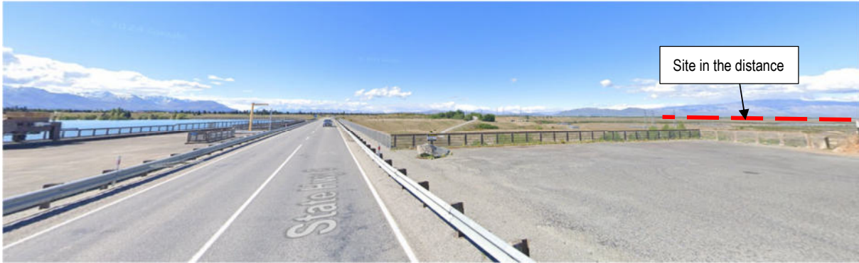
Figure 5.8: Emergent view – Northbound approaching site (Source: Google Streetview Jan 2021)
