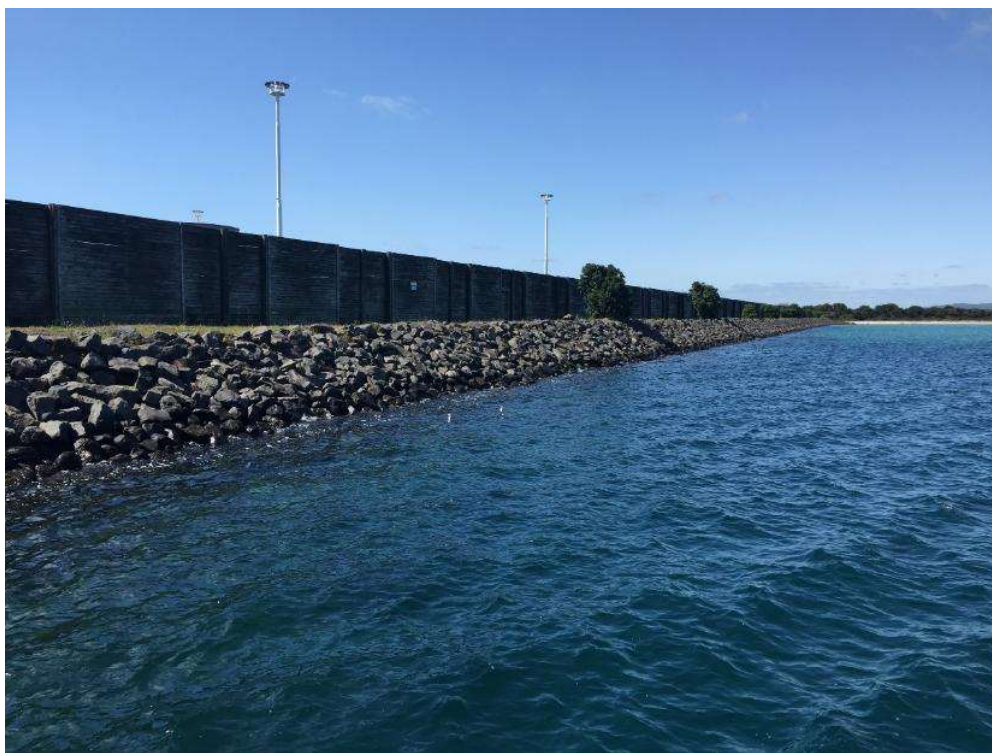
Photo 7: Riprap revetment along Northport western boundary
