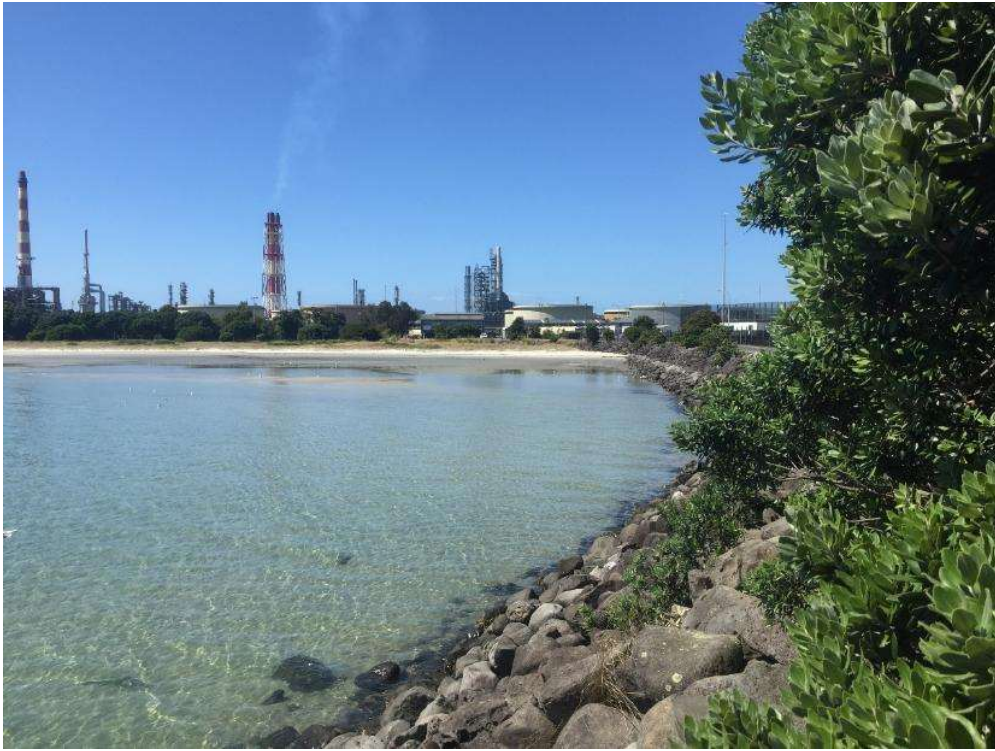
Photo 5: View of the riprap revetment along the eastern boundary of Northport boundary
