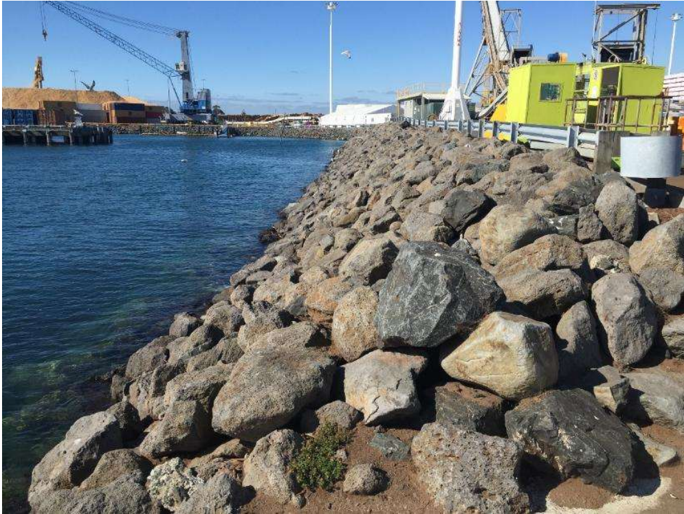
Photo 6: Riprap along the edge of Berth 3
