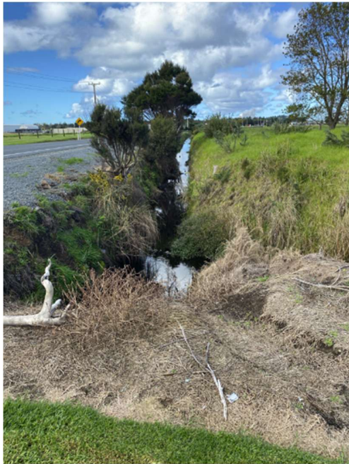
Photo 1: Roadside drain on opposite (western) side of road to the proposed car park
