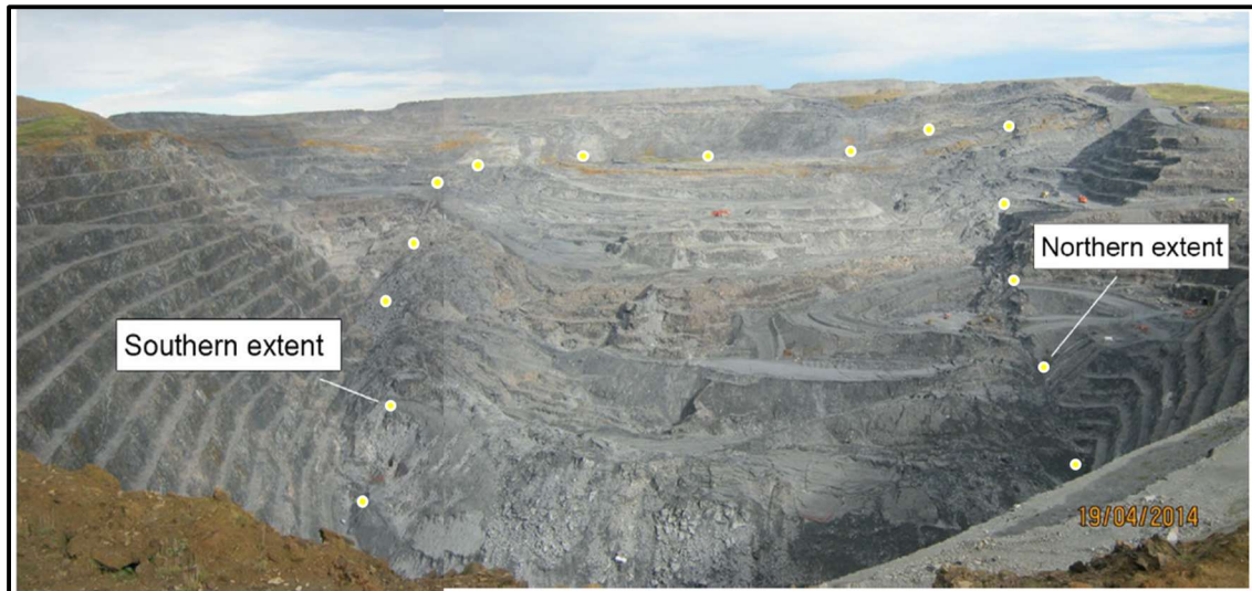
Figure-4: Photo-mosaic showing approximate outline of 2014 collapse of West Wall of Frasers Open Pit, Macraes Mine, Otago). The slide mass was estimated to be 20Mm 3 (Modified from PSM Consult Pty, 2024a)
