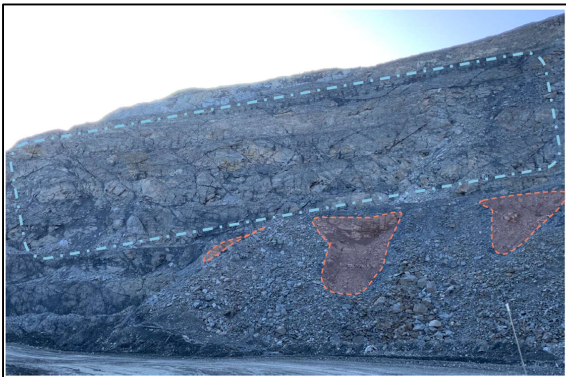
Figure-5: North Wall of Frasers Open Pit, Macraes Mine, Otago. Caving of near-surface stopes highlighted (orange). Dilated structures associated with rock-mass relaxation visible above (blue). The rock mass is expected to maintain elevated secondary permeabilities along dilated geological structures and open or caved stopes. (After PSM Consult Pty, 2024a)
