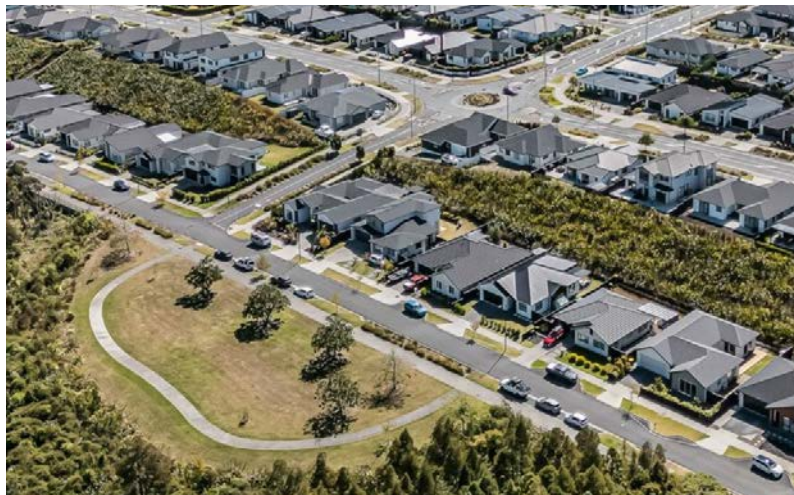
Landscaped Reinforced Earth (RE) Slopes have been used to help manage topographical changes across the development to date.
