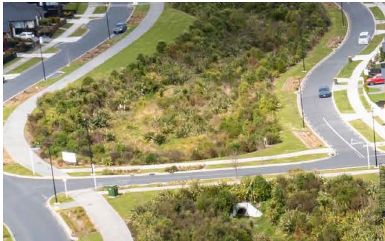
Generous riparian margins have been established and extensively revegetated to support stormwater, ecological and amenity outcomes.
