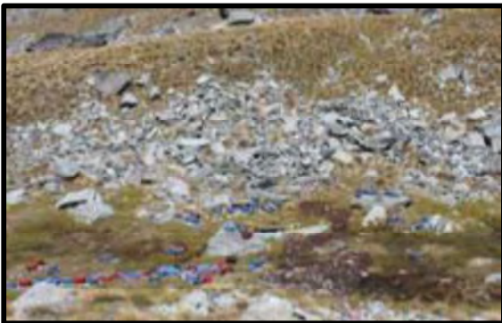
Figure 81. Cut squares of vegetation are carefully Removed in baskets and placed on wet ground Below (red & green baskets).
