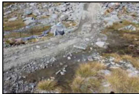
Figure 82. Same area after trench dug, pipeline laid and buried. To orient oneself note large rock upper centre left. Lower centre in Fig. 81.
