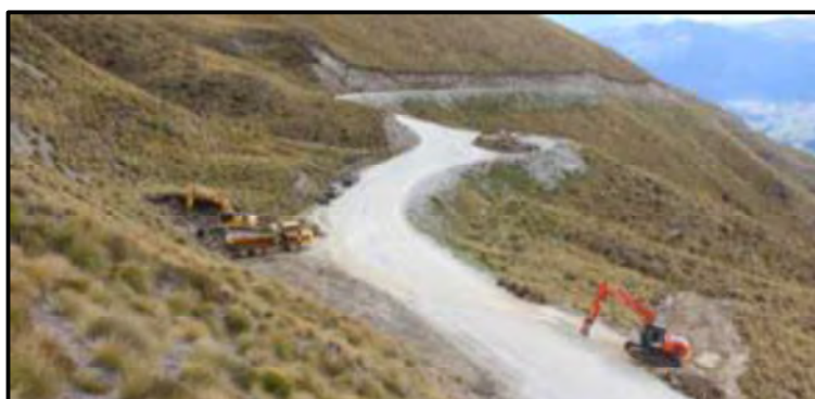
Figure 76. Further rehabilitation taking place in 2020 on the same site as Figure 75 above but the opposite view, here looking down the site. In foreground tussock clumps are being placed by digger and lower on the corner, seen as bare ground in figure 75. Later hand work is carried out to ensure plants are upright and well bedded in.
