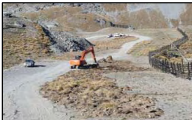
Figure 76. Further rehabilitation taking place in 2020 on the same site as Figure 75 above but the opposite view, here looking down the site. In foreground tussock clumps are being placed by digger and lower on the corner, seen as bare ground in figure 75. Later hand work is carried out to ensure plants are upright and well bedded in.
