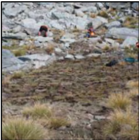
Figure 83. After two months all vegetation that had been removed was relocated and placed like a patchwork quilt, over the reformed ground and packed into place.
