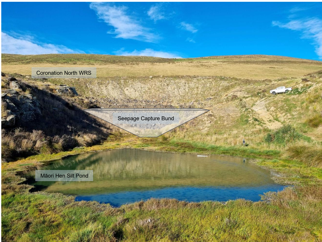
Figure F-2.8 Māori Hen Silt Pond, looking south towards Coronation North WRS, showing location of discrete toe seepage and proposed toe bund
