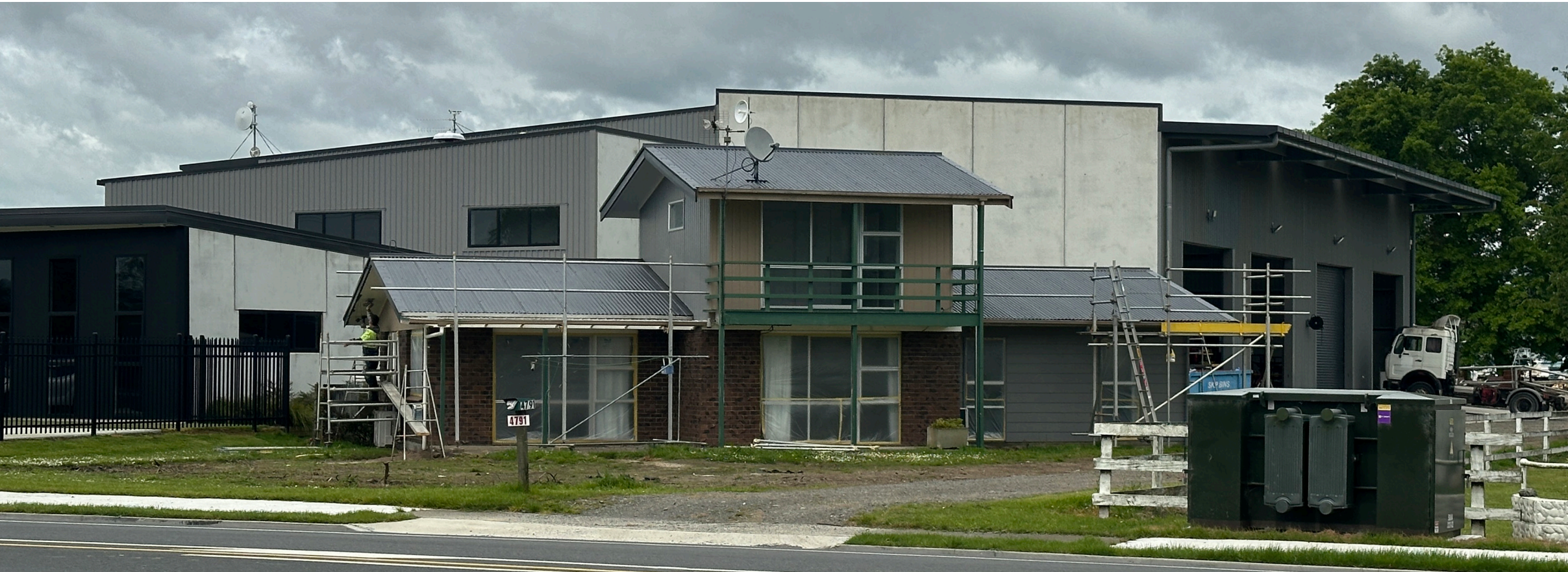
Photo 2 (0825): Image taken from 4791 State Highway 29 looking southeast
