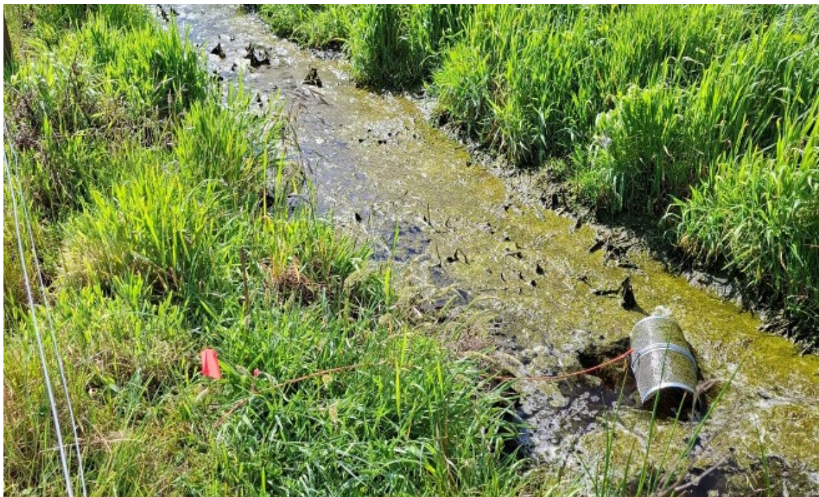
Figure 13. Drain condition example (ecoLogical Solutions).
