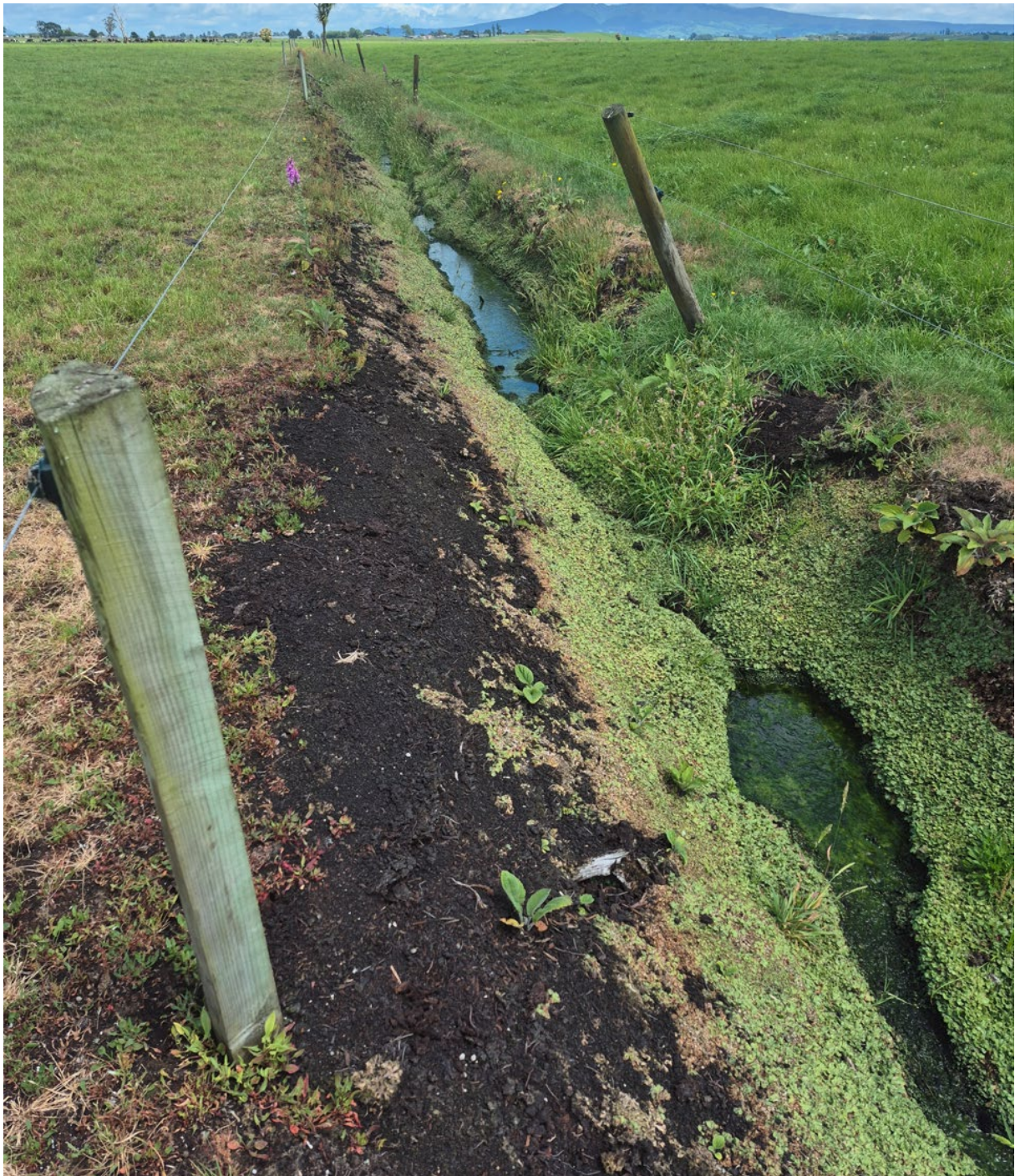
Figure 5: Central Farmland Drain Within the Industrial Area (WGA Field Visit, 11 November 2025)
