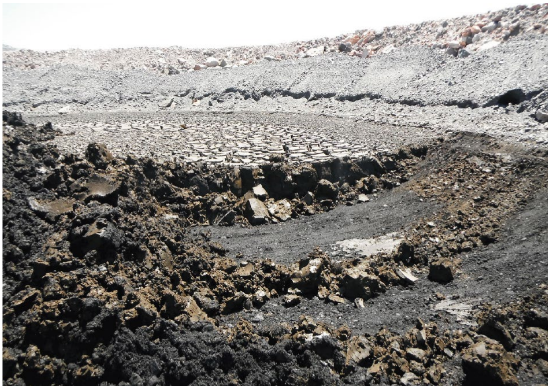
Figure 21: Stockton AMD sludge filter beds.
