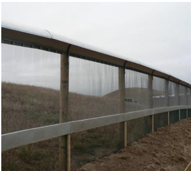
Figure 9. A pest exclusion fence (as constructed by Pestproof Fences Ltd).
