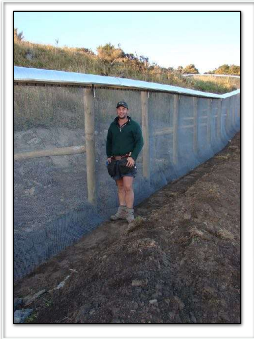
Fig. 6.: A galvanised Pestproof Ltd exclusion fence that is nearing completion. The trench containing the buried skirt is about to be back filled - the last job in the construction process. This type of fence is as simple as a pest-proof fence can get. It is essentially a continuous wall of woven mesh, supported by capping and posts. It has no stapled mesh overlaps, above or below ground, which can potentially open up and become entry points for pests over time. This feature is essential for the long-term exclusion of mice.
