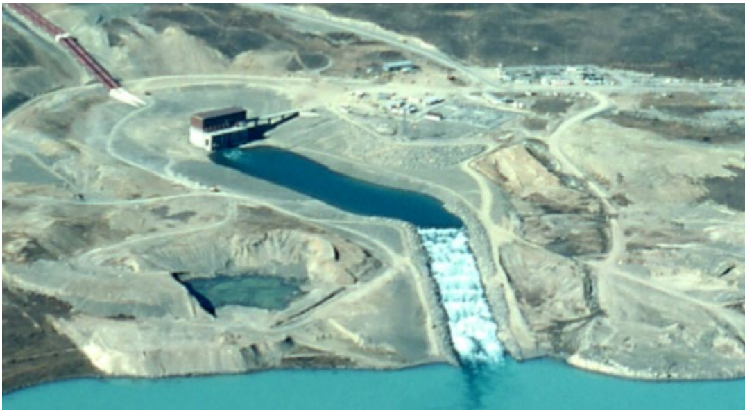
Figure 20 Lake Pūkaki at 504.3 m RL showing the full extent of the tailrace and weir.
