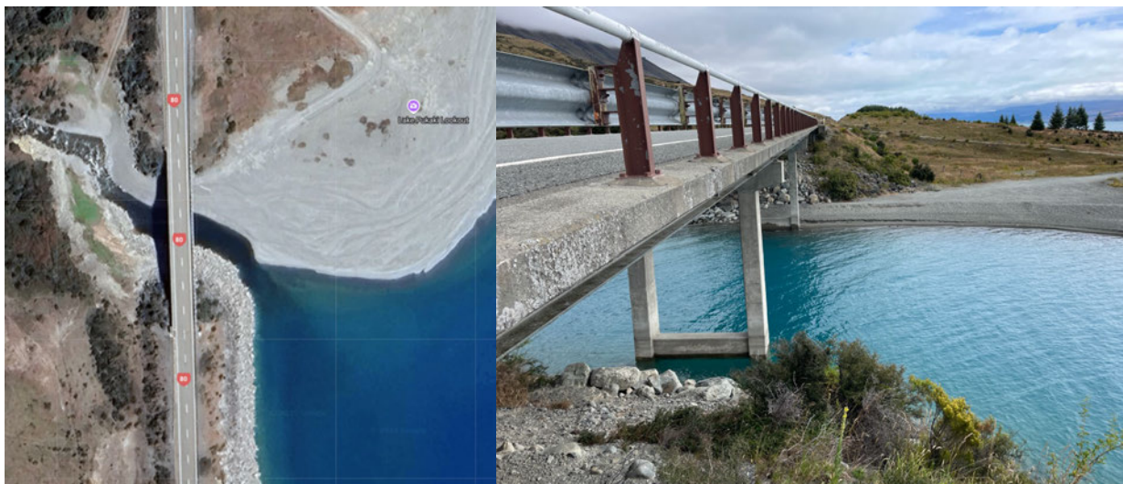
Figure 24 Left: Aerial view of Boundary Stream Bridge (SH 80 RS 17 RP 12.64 – 12.7, Source: Google Maps). Right: Site visit photo showing the partially submerged bridge abutments.
