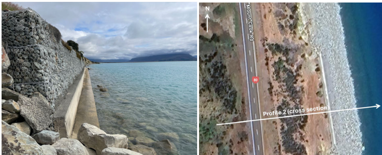
Figure 23 Left: Photo taken of the gabion retaining wall facing north. Right: Aerial image of the Gabion retaining wall between SH 80 RS 17 RP 12.64 – 12.7 (Source: Google Maps).
