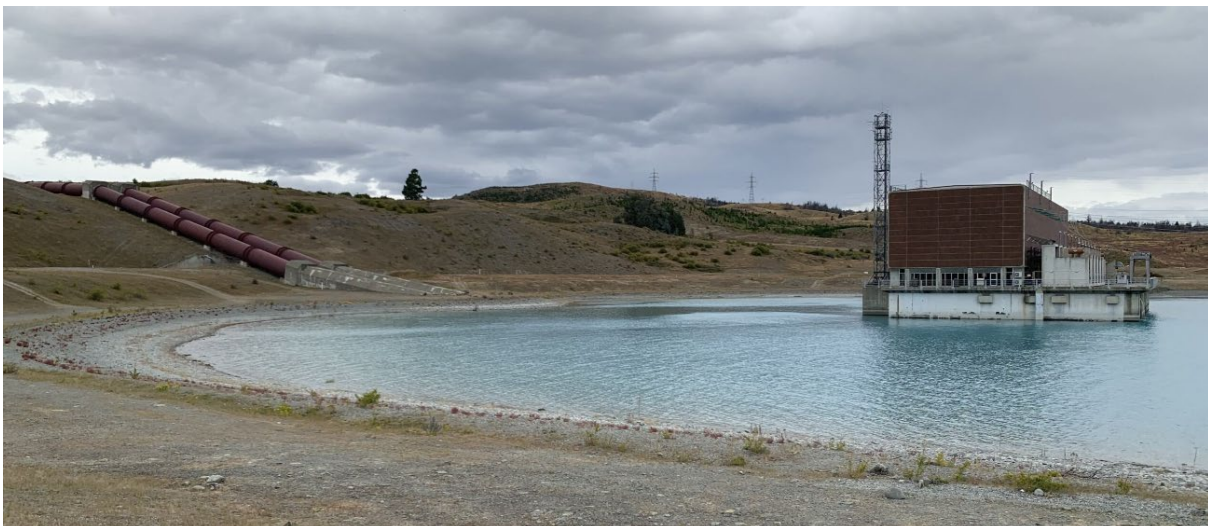
Figure 18 Site visit photo of Tekapo B Power Station showing the two penstocks.
