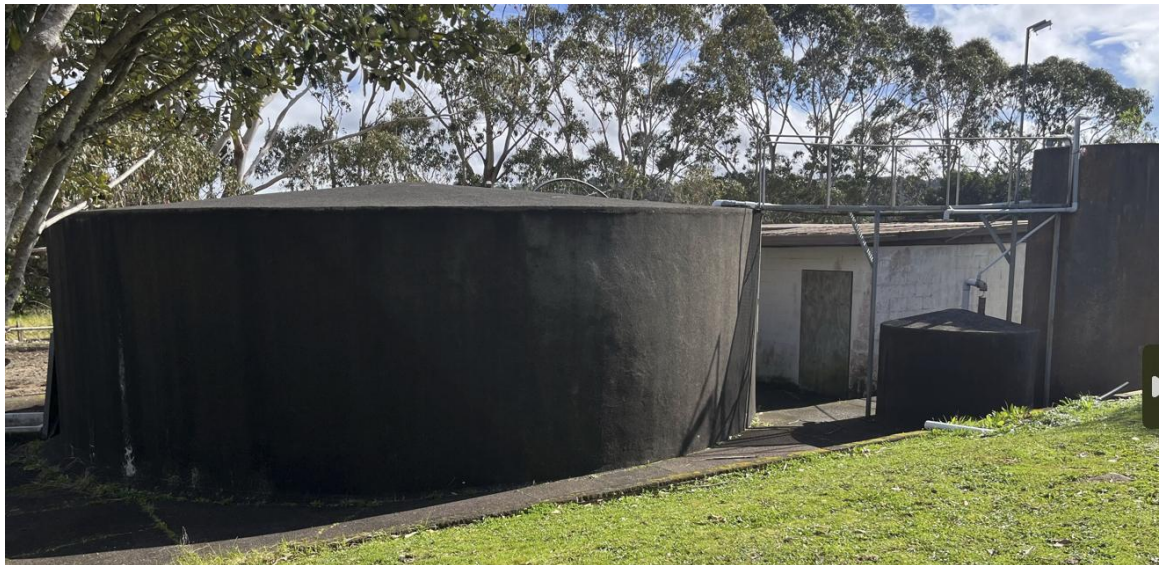
Figure 47. Photograph showing the water tank beside the community hall, looking northwest
