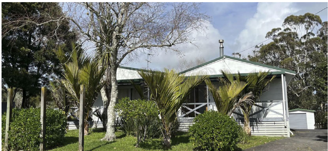
Figure 46. Photograph showing the community hall at 505 Paremoro Road, looking south
