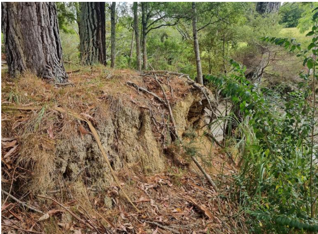
Figure 31. Photograph showing exposed section of eroded creek bank in Area 2
