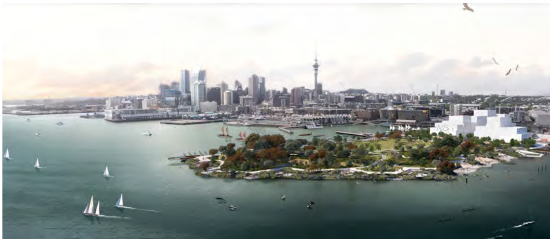
Figure 7: The vision for Te Ara Tukutuku. The site at 188 Beaumont Street and the Orams Marine Village land can be seen in the far right of the image located behind the indicative 'white card' massing of future development within Te Ara Tukutuku enabled by the Precinct provisions (source: A new public space for the people of Tāmaki Makaurau. - Auckland Council www.audo.co.nz/projects/tearatukutuku/#concept-design )
