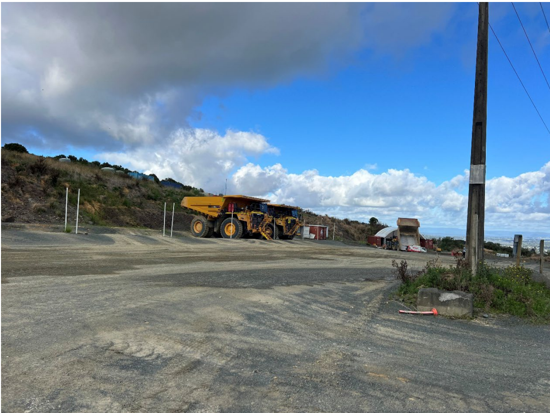
Photograph 8: Looking southwest at heavy machinery and the half-dome vehicle maintenance structure at C+R Rack.
