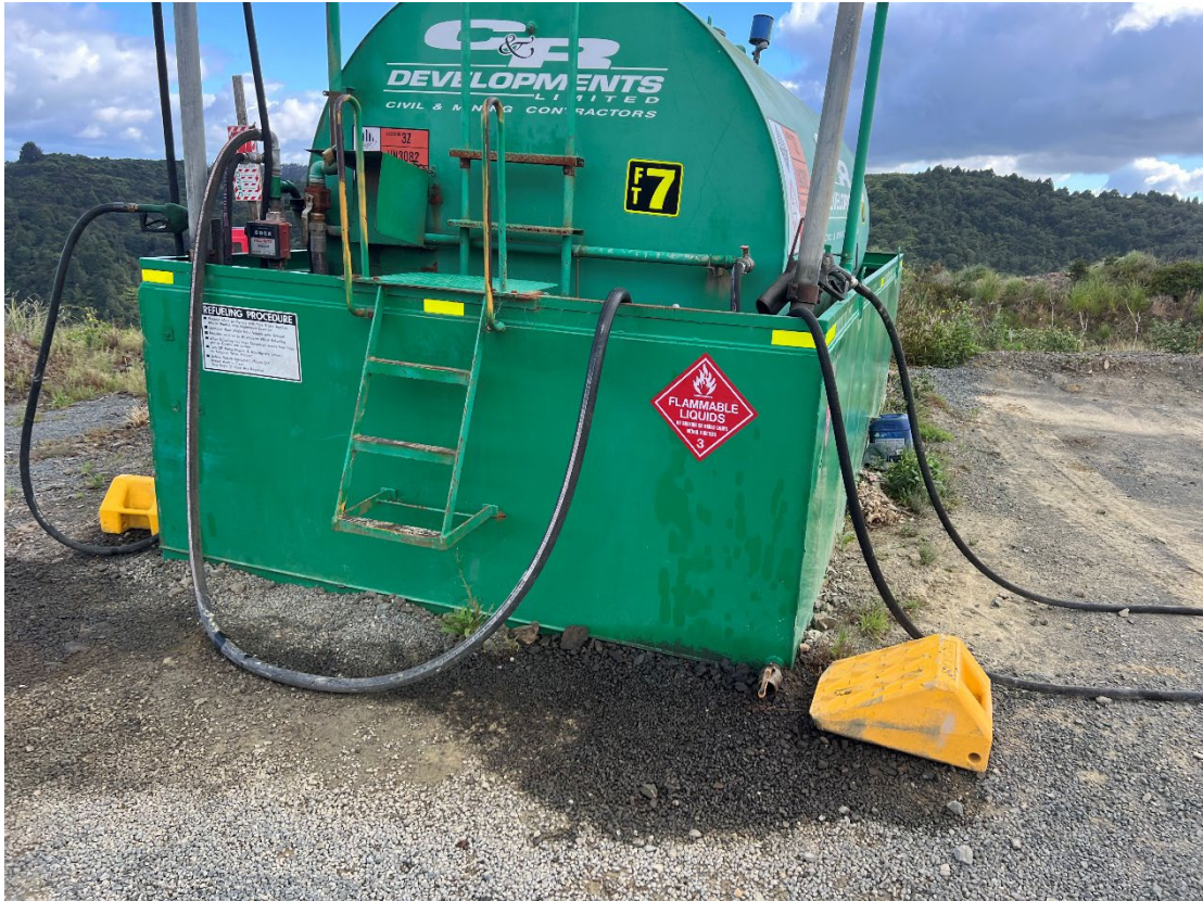
Photograph 11: Looking northeast at the western AST with hydrocarbon staining on the ground where PMS13 was taken.
