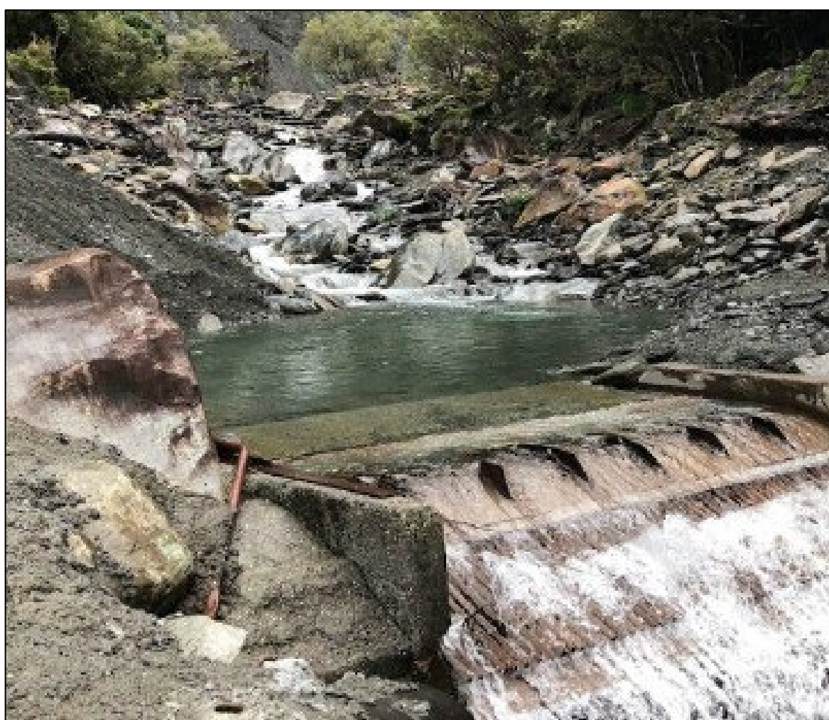
Figure 3: Example of a Tyrolean weir (Source: Stantec, 2025).
