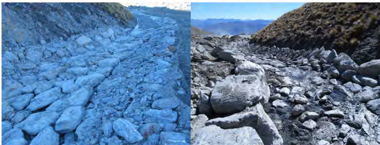
Figure 3. Rastus Burn Creek Stream Training and Armouring
