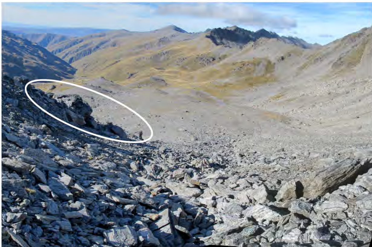
Figure 37. Potentially unstable rocks viewed from immediately below the ridge line
