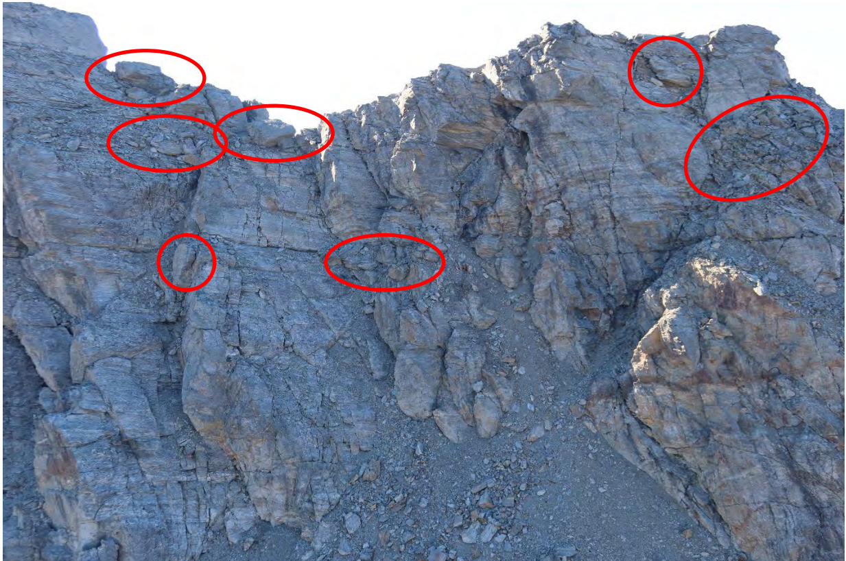
Figure 40. Locations of potentially unstable rock along the ridgeline
