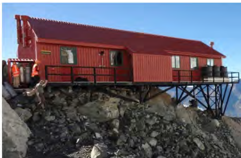
Figure 29. Plateau Hut on Aoraki Mt Cook with a combination of structural design and architectural detailing for wind such as the vestibule over the door
