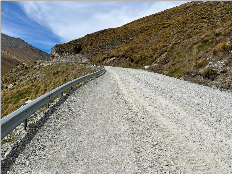
Photograph 4-3: Typical gravelled section of Remarkables Ski Field Access Road (Source: Stantec)
