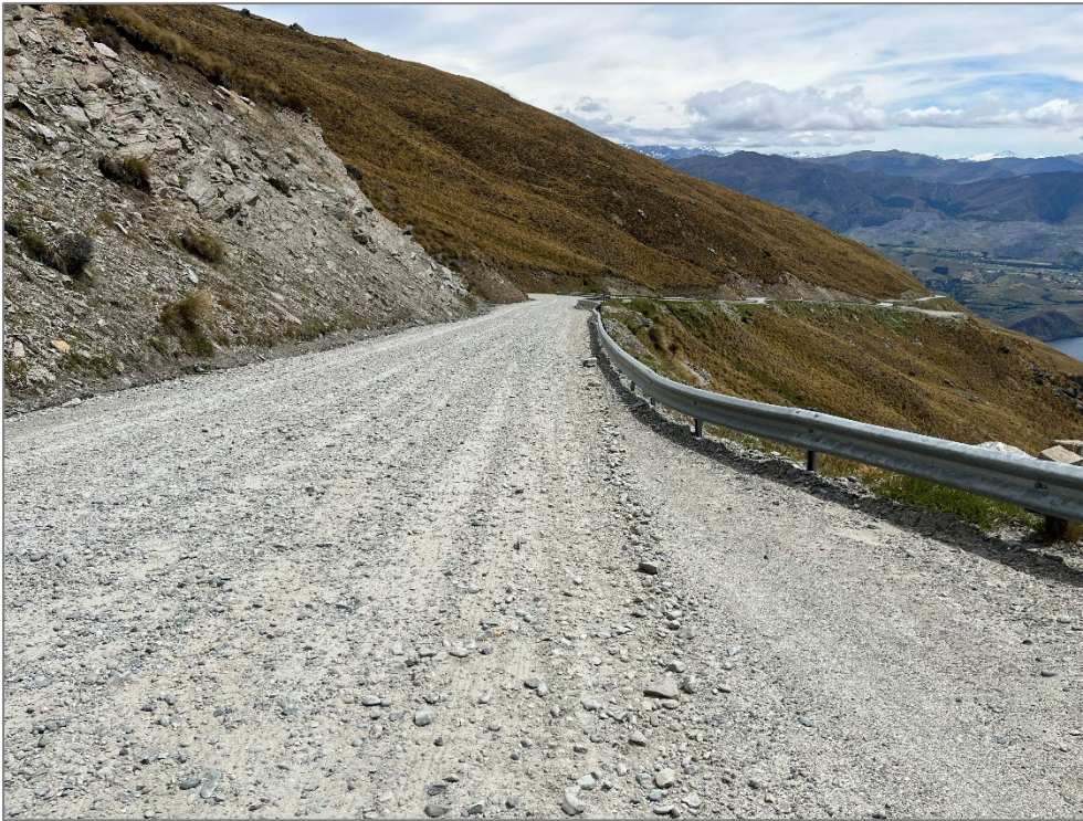
Photograph 4-4: Typical gravelled section of Remarkables Ski Field Access Road (Source: Stantec)
