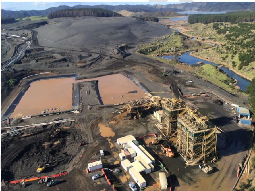
Figure 1. Spiral Plant and SSP Ponds.
