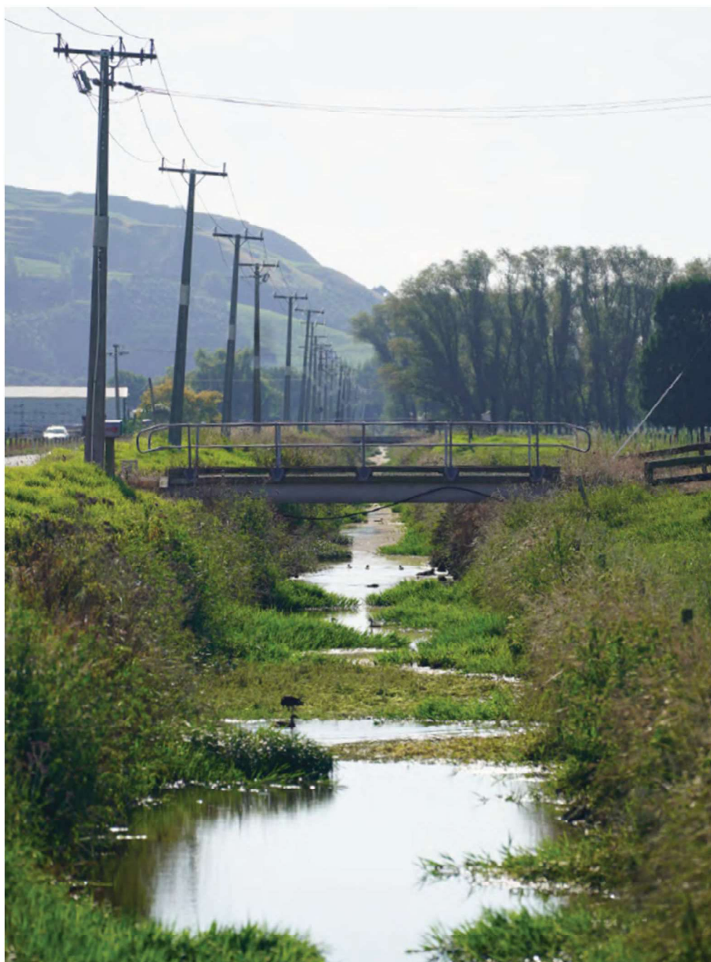
Figure 10 - The Bell Road Drain, Looking West (Source: Maven)
