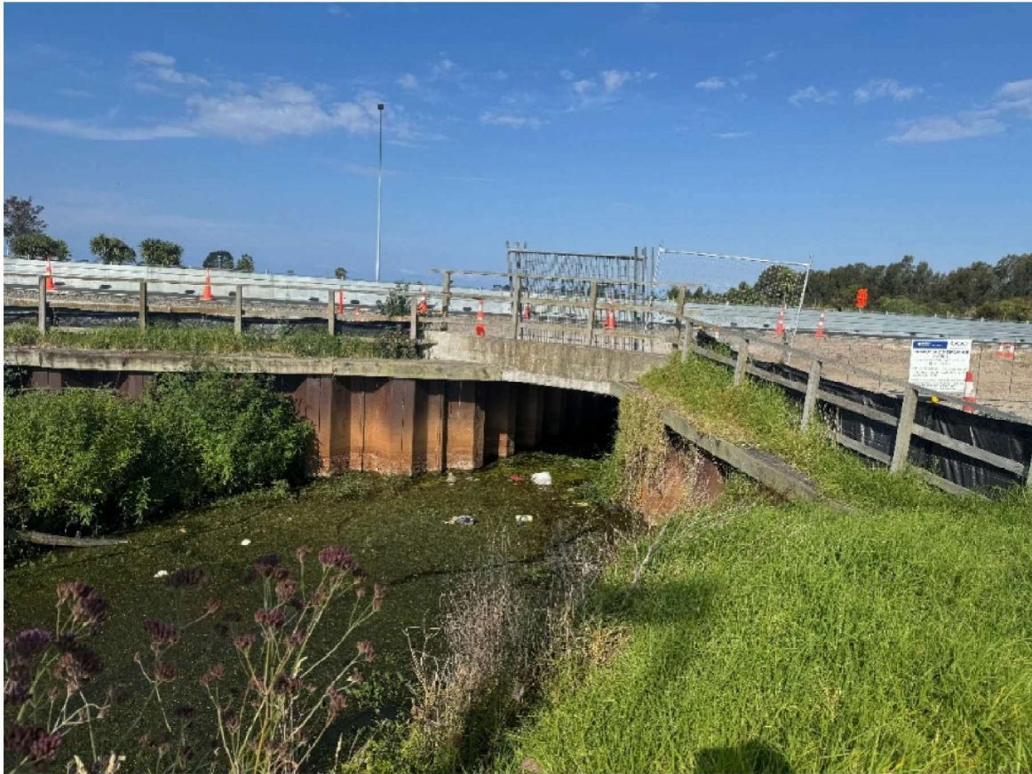
Figure 11 - The Bell Road Drain TEL Culvert, Looking Northeast (Source: Maven)
