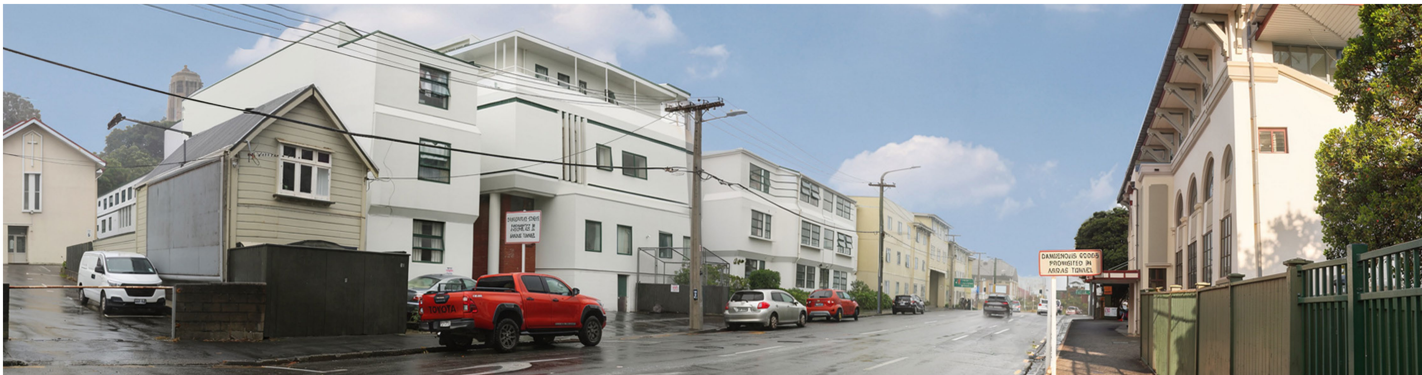
VP7 | SUSSEX STREET LOOKING NORTH | EXISTING VIEW
