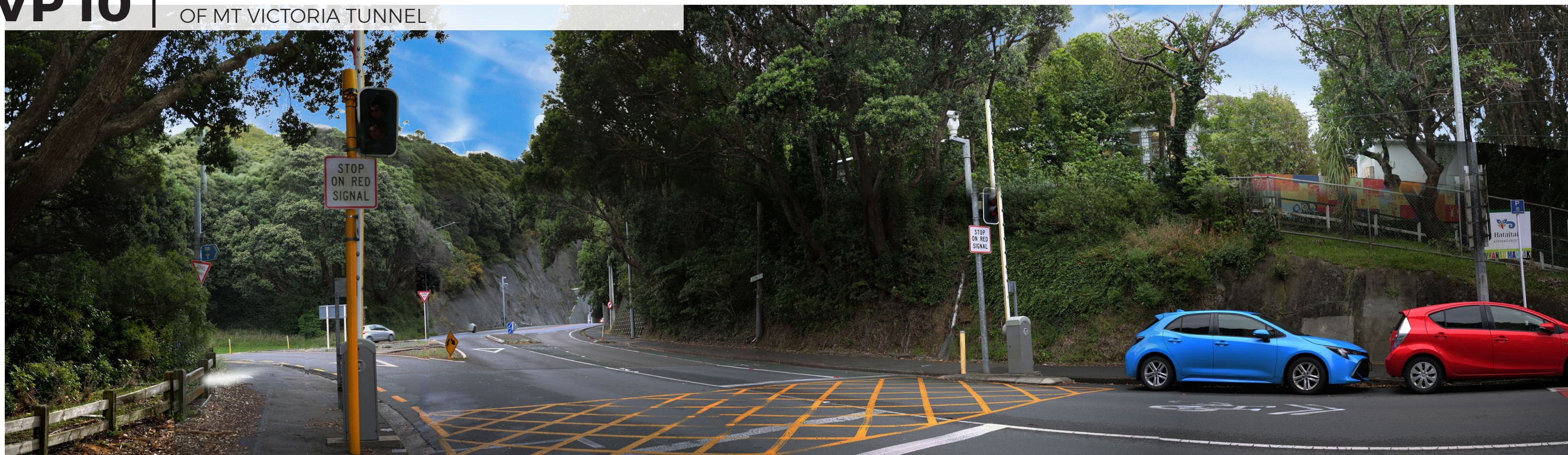
VP10 | TAURIMA STREET LOOKING TO EASTERN PORTAL OF MT VICTORIA TUNNEL | EXISTING VIEW
