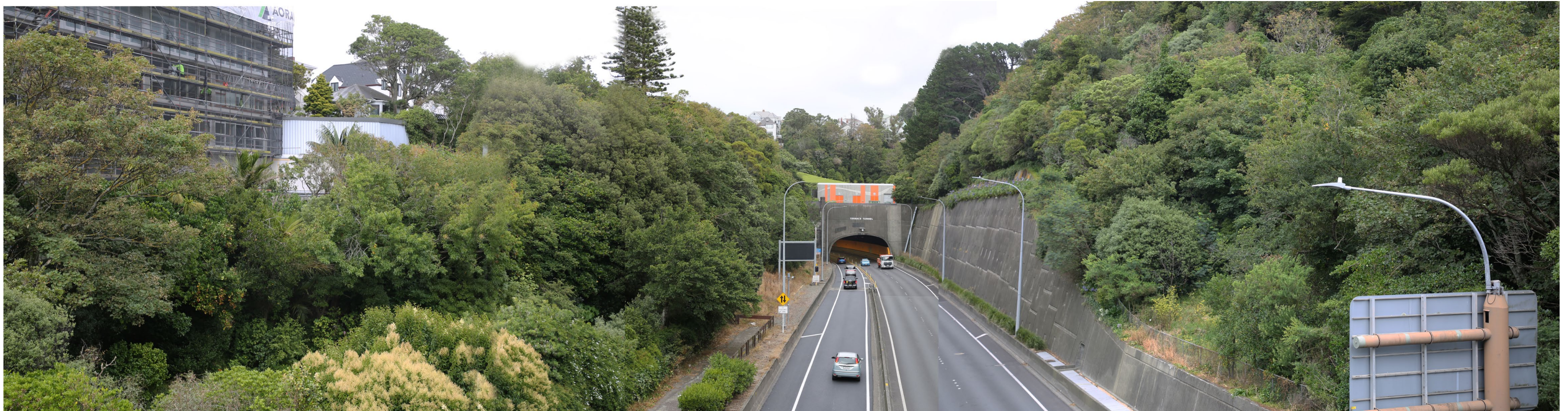
VP1 | TERRACE TUNNEL NORTH FROM x STREET | EXISTING VIEW
