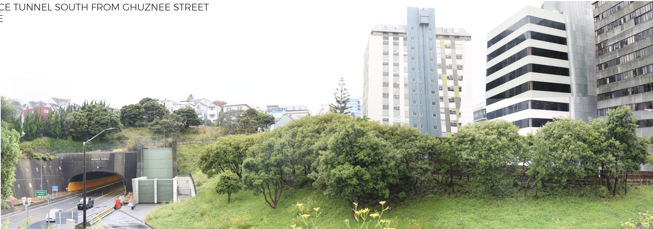
VP2 | TERRACE TUNNEL SOUTH FROM GHUZZEE STREET BRIDGE | EXISTING VIEW
