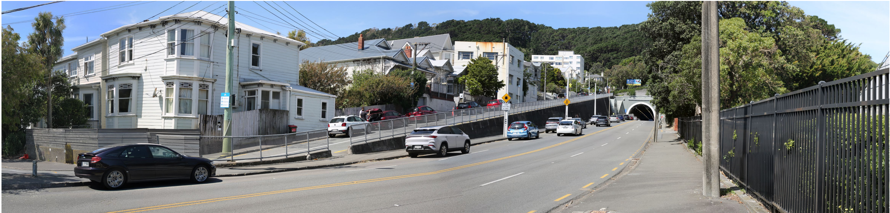
VP9 | PATERSON STREET LOOKING TO WESTERN PORTAL OF MT VICTORIA TUNNEL | EXISTING VIEW
