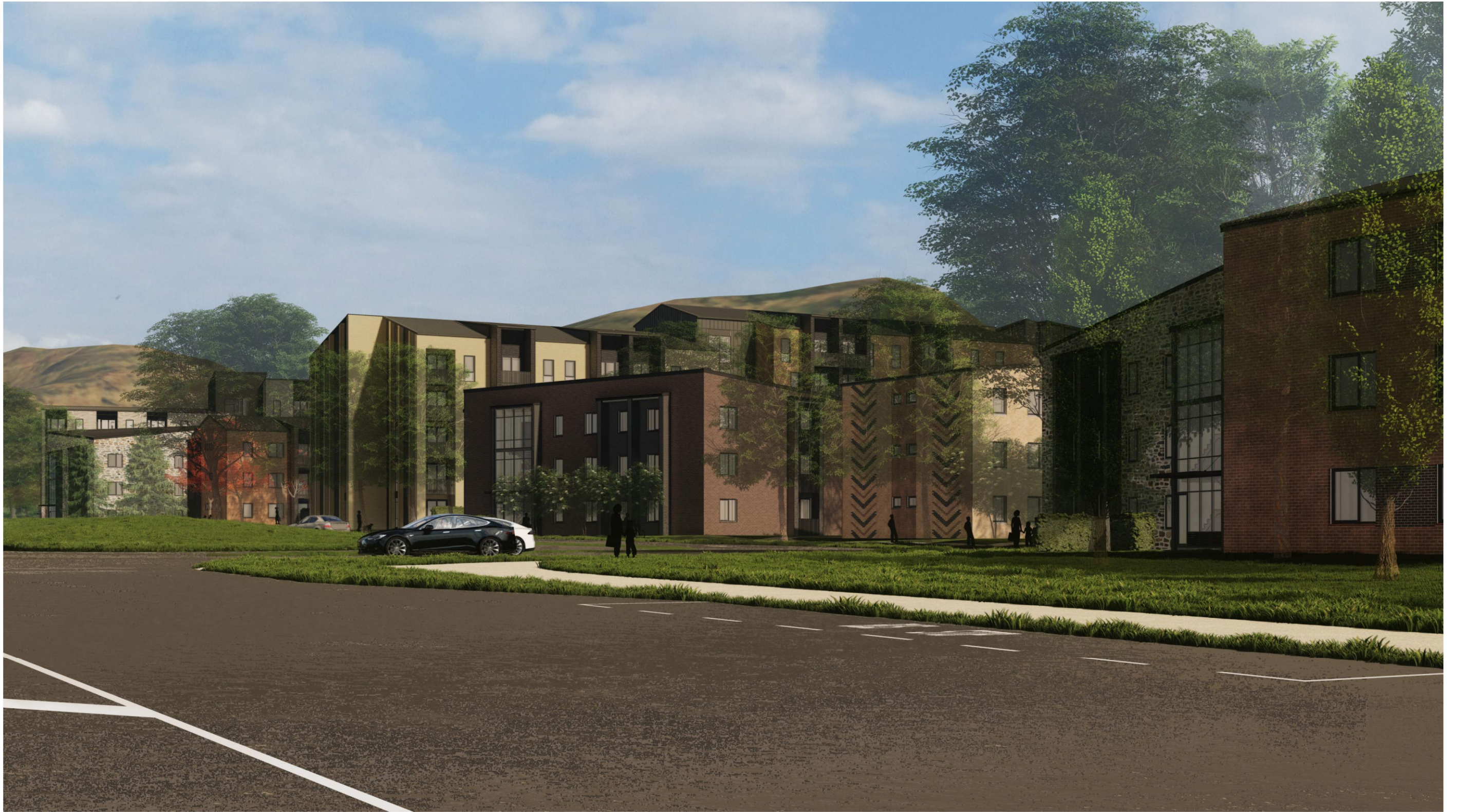
VIEW LOOKING WEST TOWARDS STATE HIGHWAY 6 AND LOWER SHOTOVER ROAD INTERSECTION
