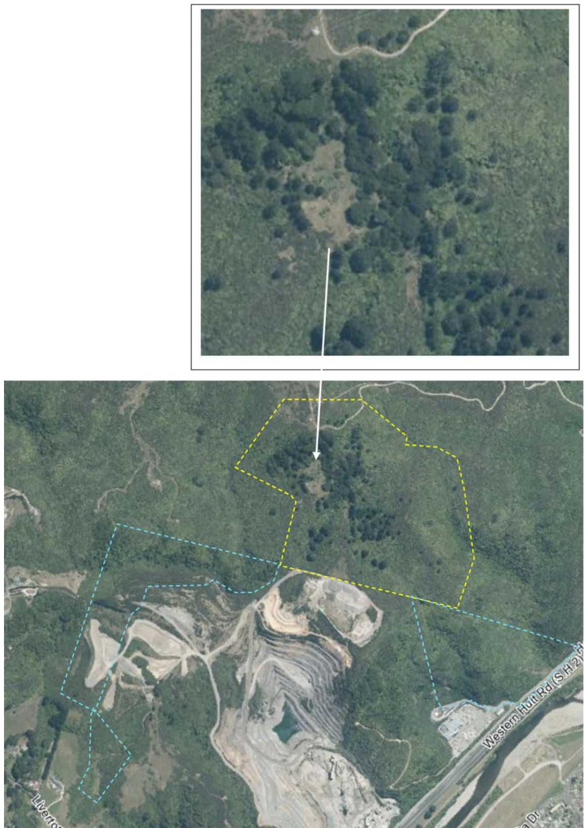
Figure 16. Aerial photograph dated 2005 showing the proposed OBDA (outlined by yellow dashed line) and three land exchange areas at the Belmont Quarry (outlined by blue dashed lines,) with detail of the area that previously contained structures shown in upper inset (source from: Google Earth)
