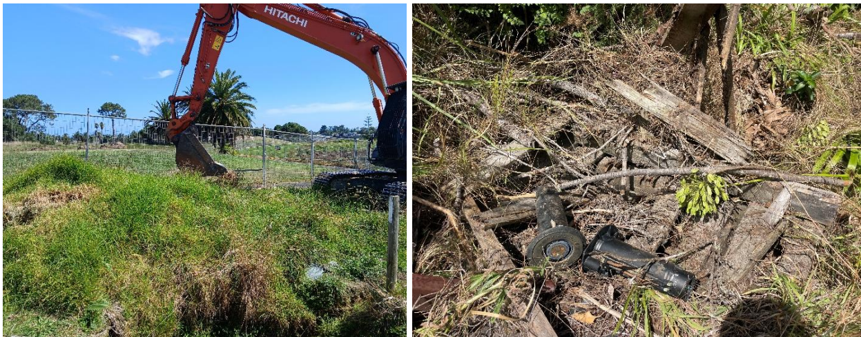
Photo 1: Machine-assisted searches utilising toothed bucket through grass habitat (left); Manmade debris which was first searched by hand (right) during lizard search and salvage
