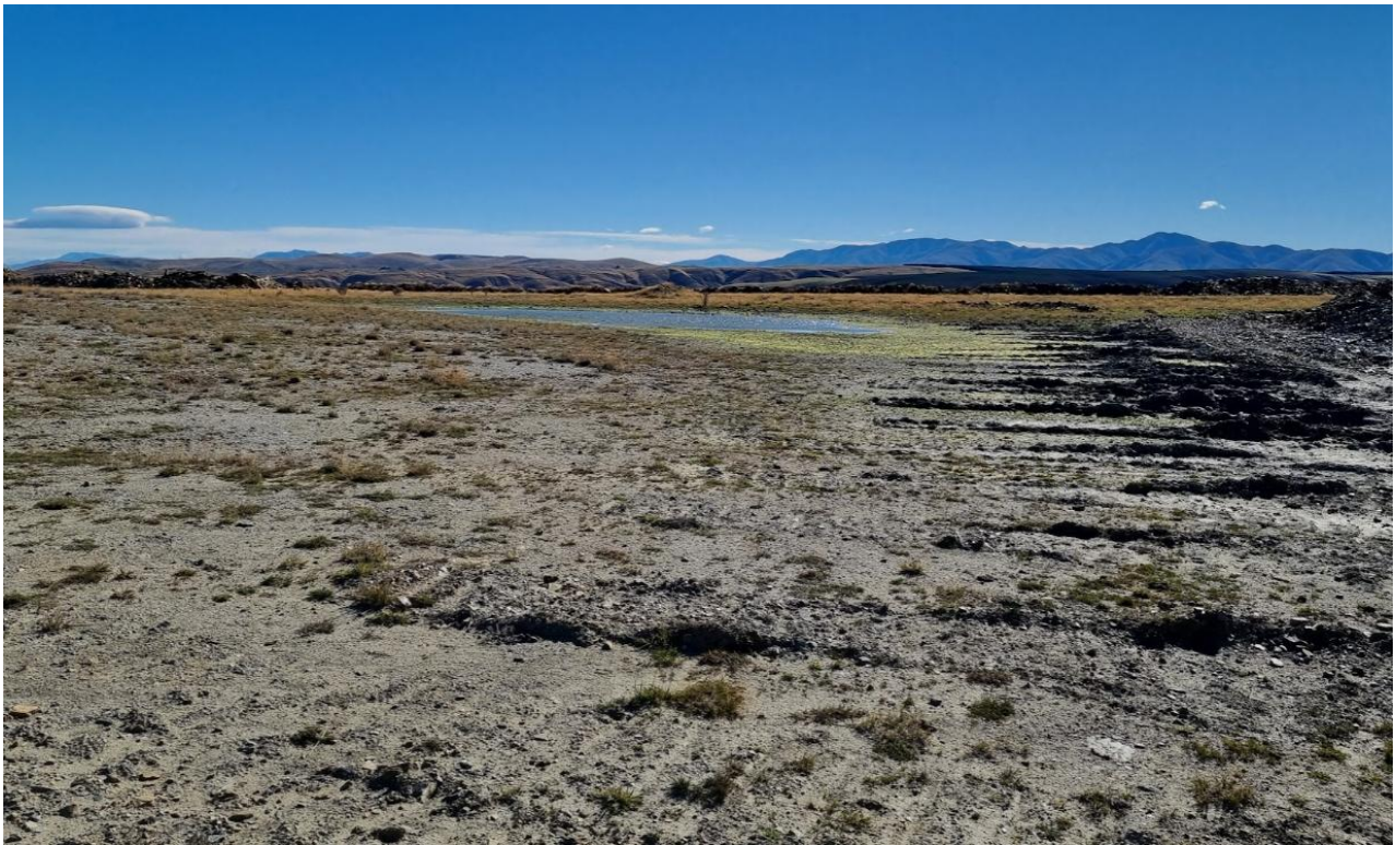
Figure G-2.10 Photo of Trimbell's WRS surface showing localised ponding
