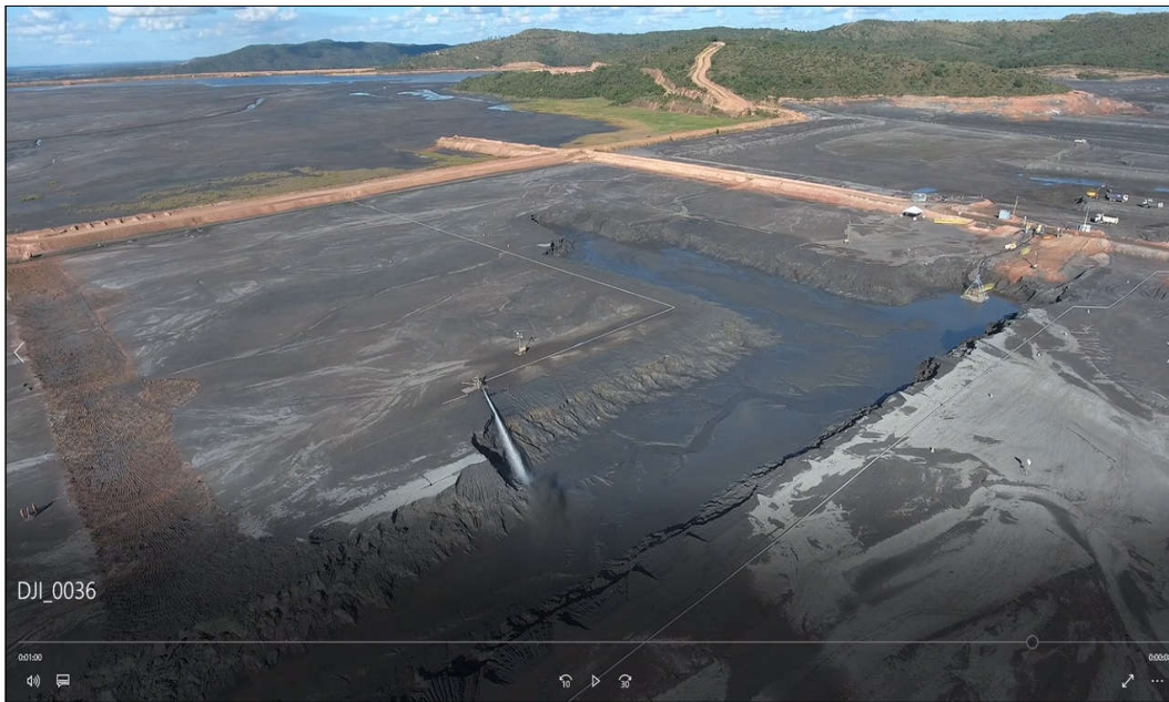
Figure 5-11 Bench and Mining Block Development during Hydraulic Mining
