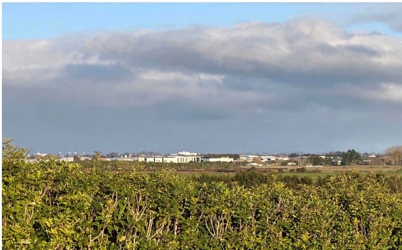
Photo 6: Example of Te Rapa Industrial Development Area with upper sections of building visible in the landscape
