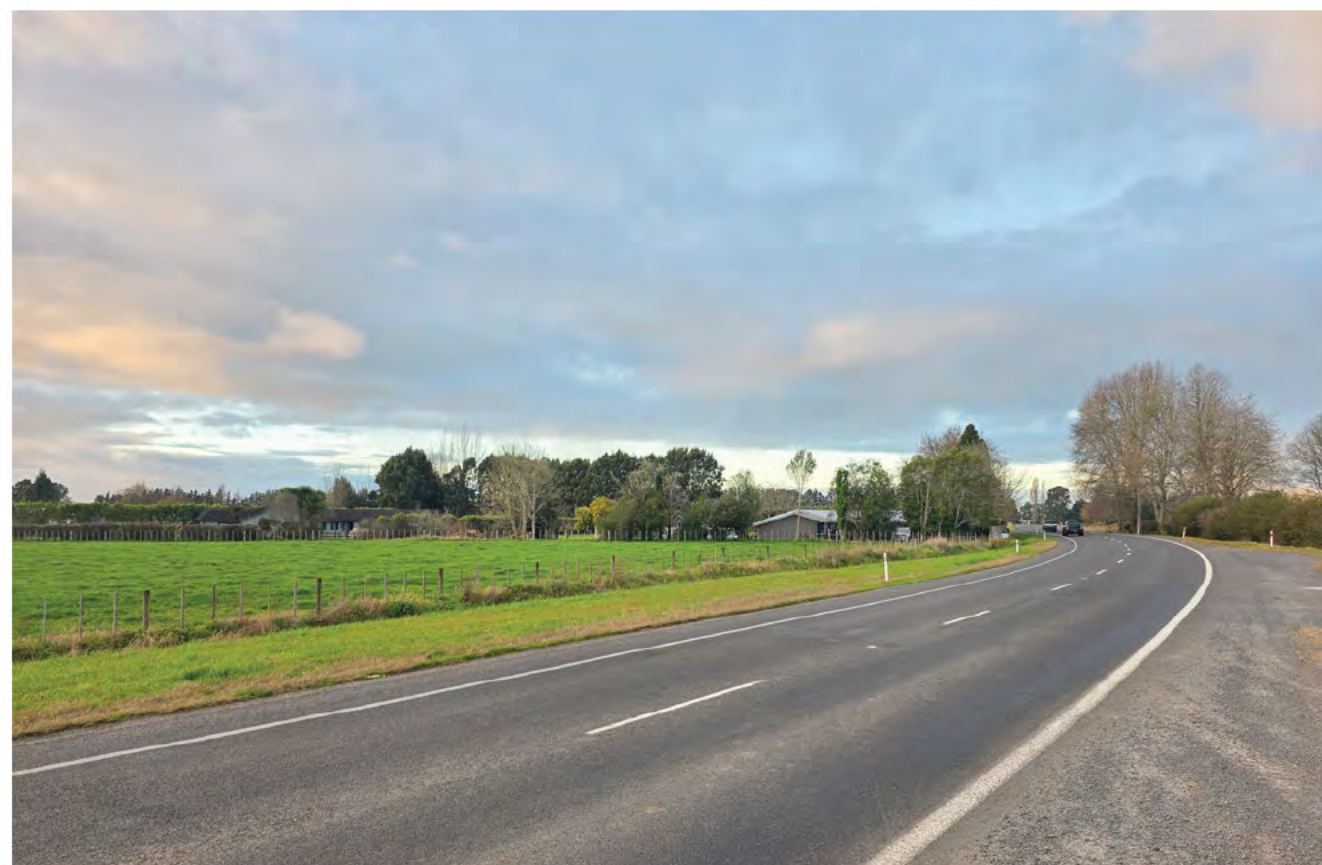
Photo PVP 3- View looking east along SH39 (adjacent to 335 SH39)
