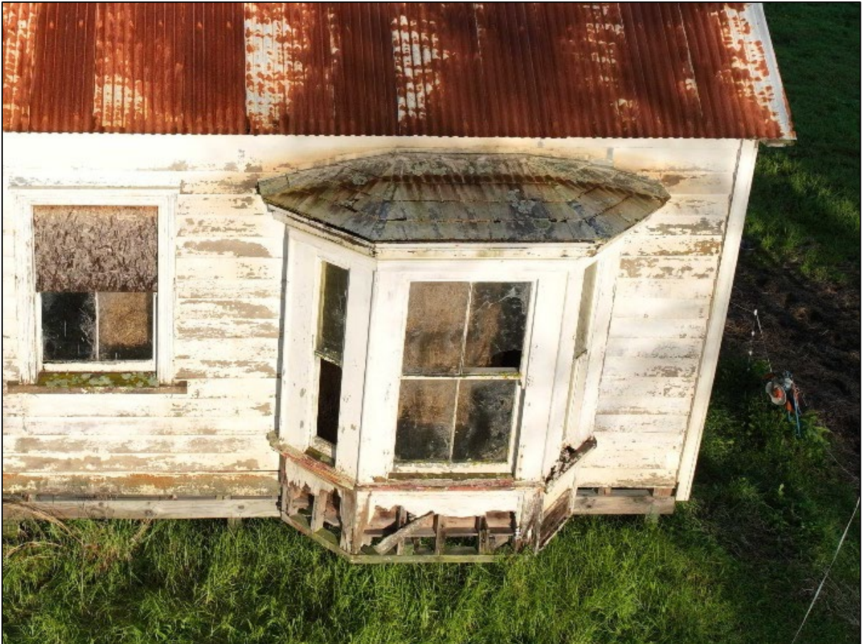
Figure 7. Bay window with shingle roof.
