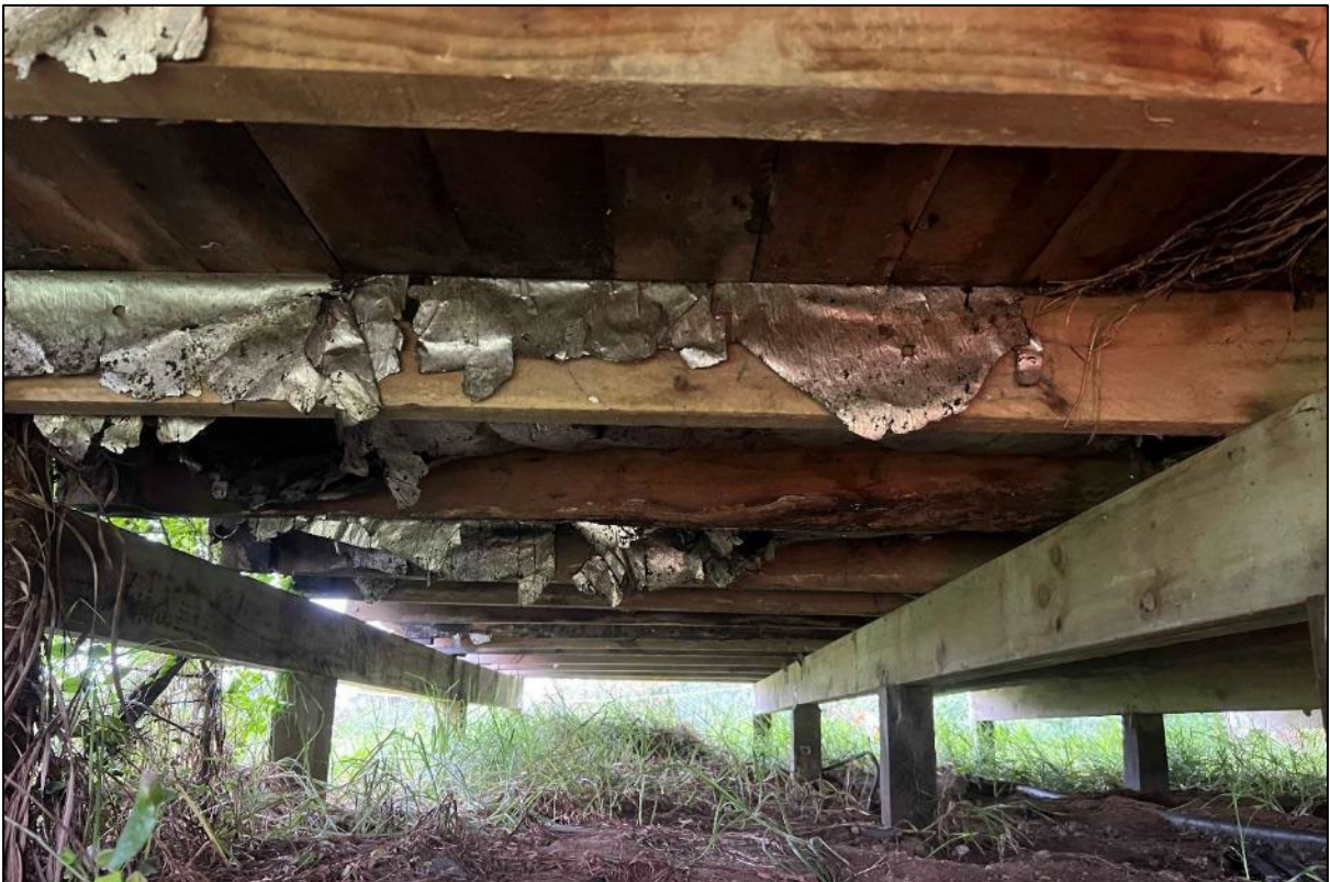
Figure 24. Subfloor image showing a mixture of new and old joists and floorboards above.
