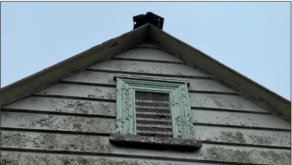
Figure 20. Louvre window on south elevation.
