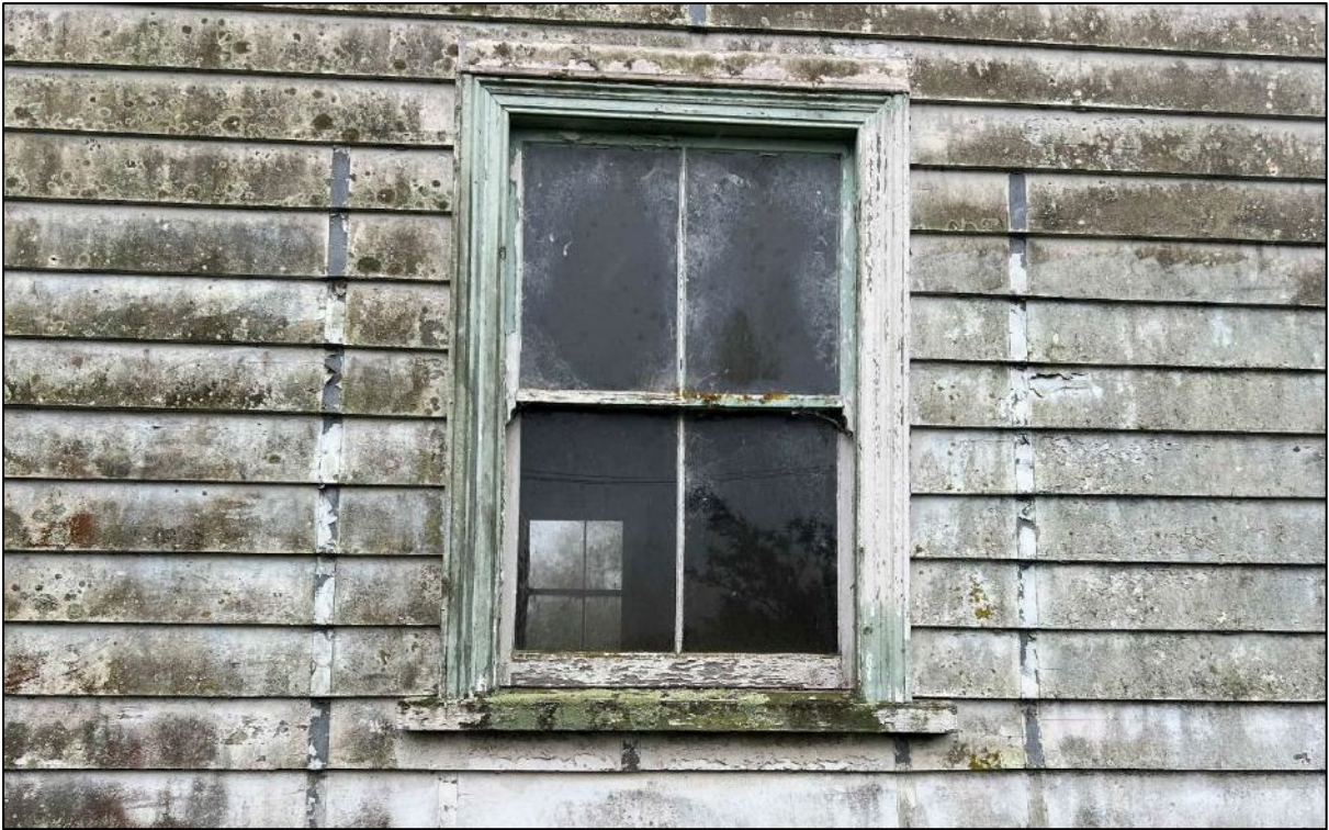
Figure 19. Window on south elevation.
