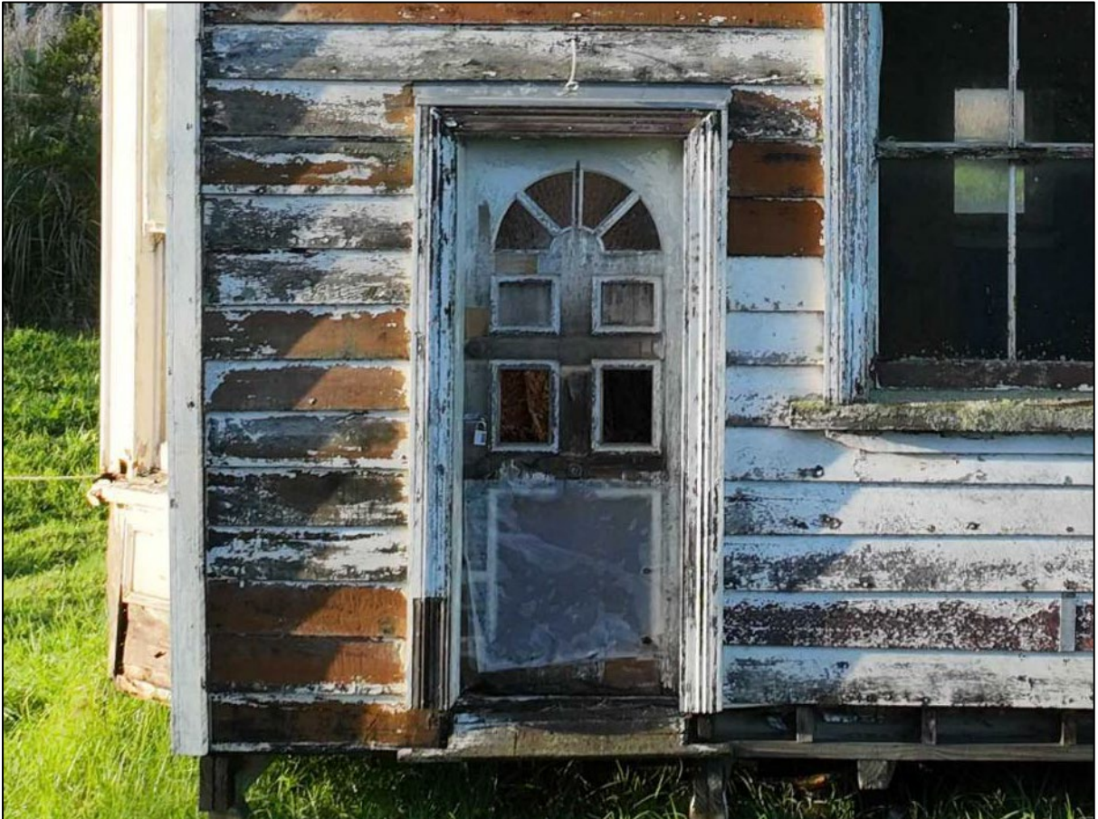
Figure 22. Door on north elevation.
