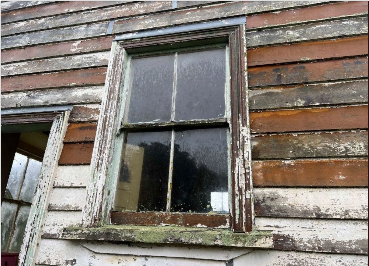
Figure 17. Window on north elevation.
