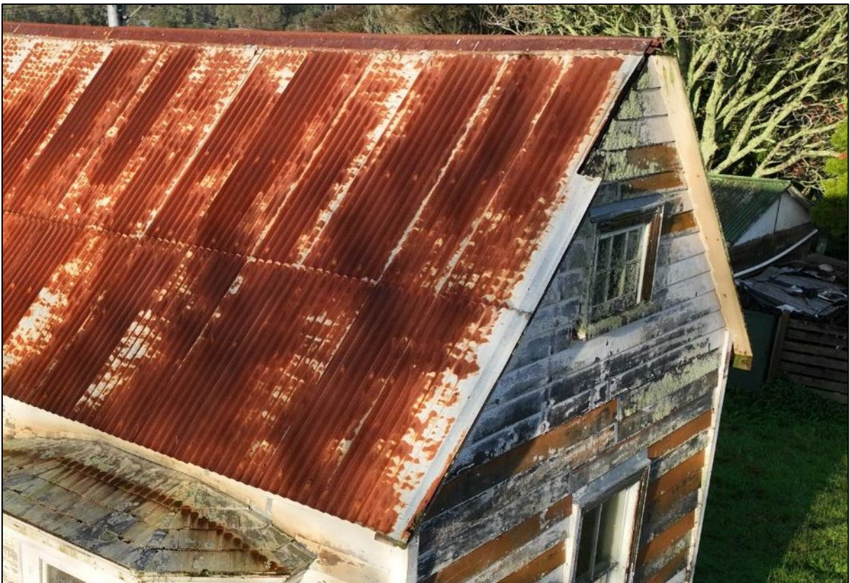
Figure 6. North elevation gable with notch cut out of roofing for former chimney.
