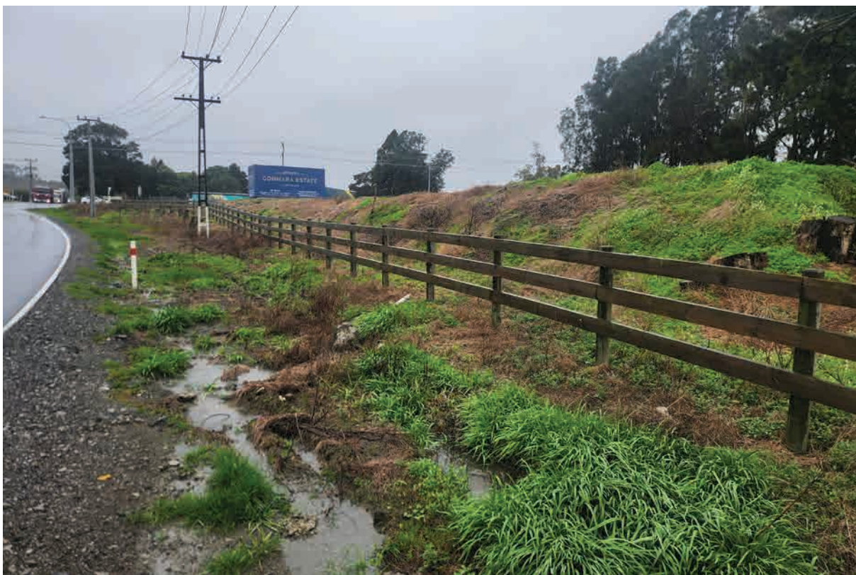
Figure 17. View east along Alfriston Road showing built up fill on 1345 Alfriston Road.
