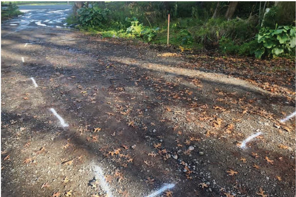
Figure 12. View south across driveway of 242 Redoubt Road showing built up surface.
