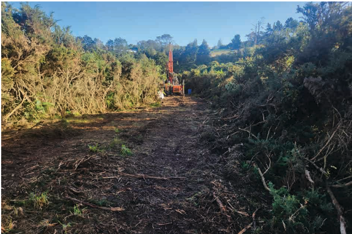
Figure 13. View north of a mown track through gorse for drill rig access.
