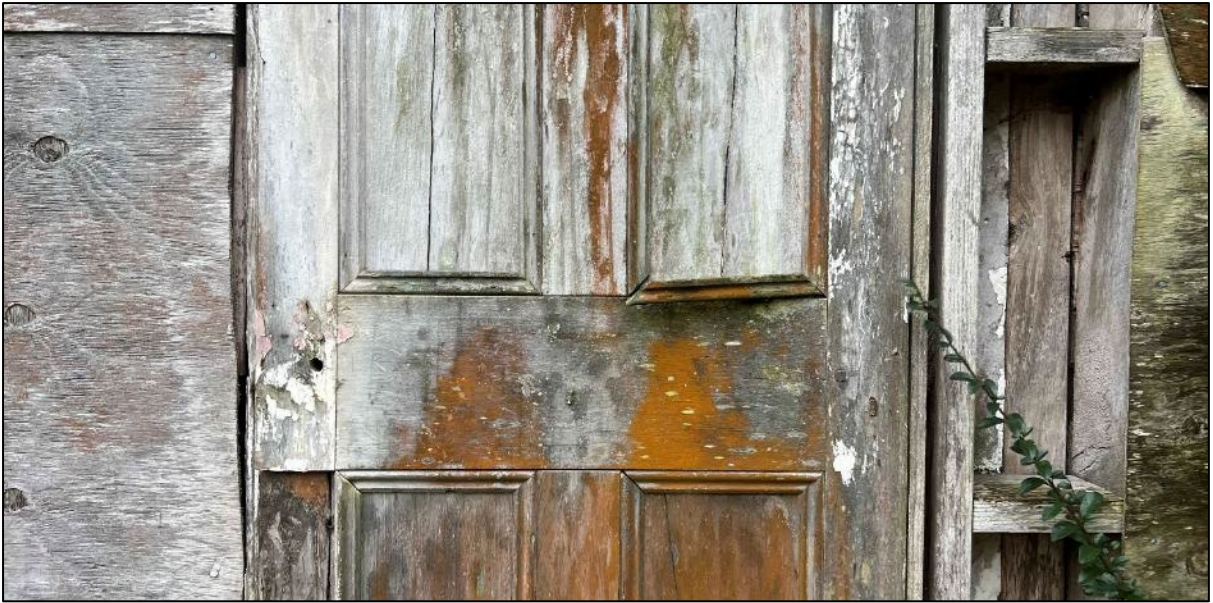
Figure 21. Detail showing biogrowth, splitting, and loose bolection moulding.
