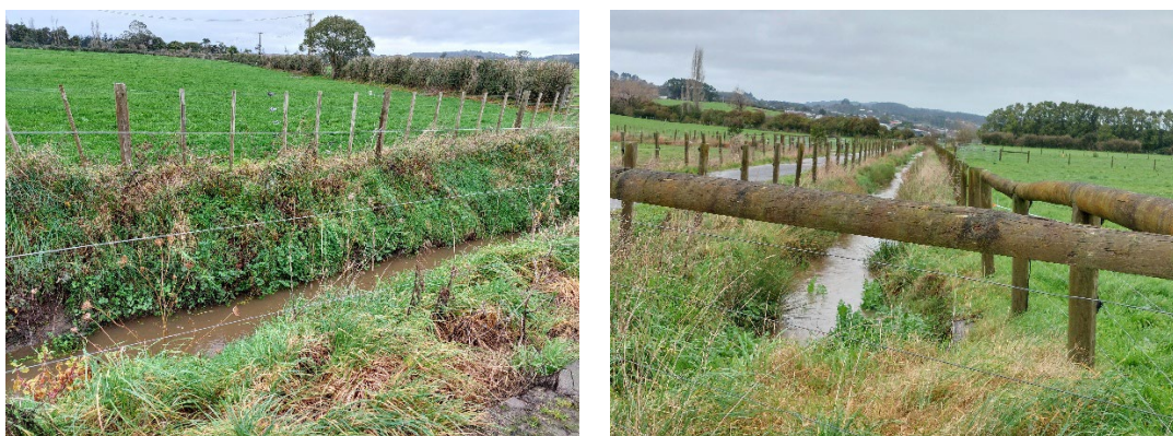
Figure 2: Drains observed flowing well at the site visit, during wet conditions. Photos: R Underwood 11 July 2025.
