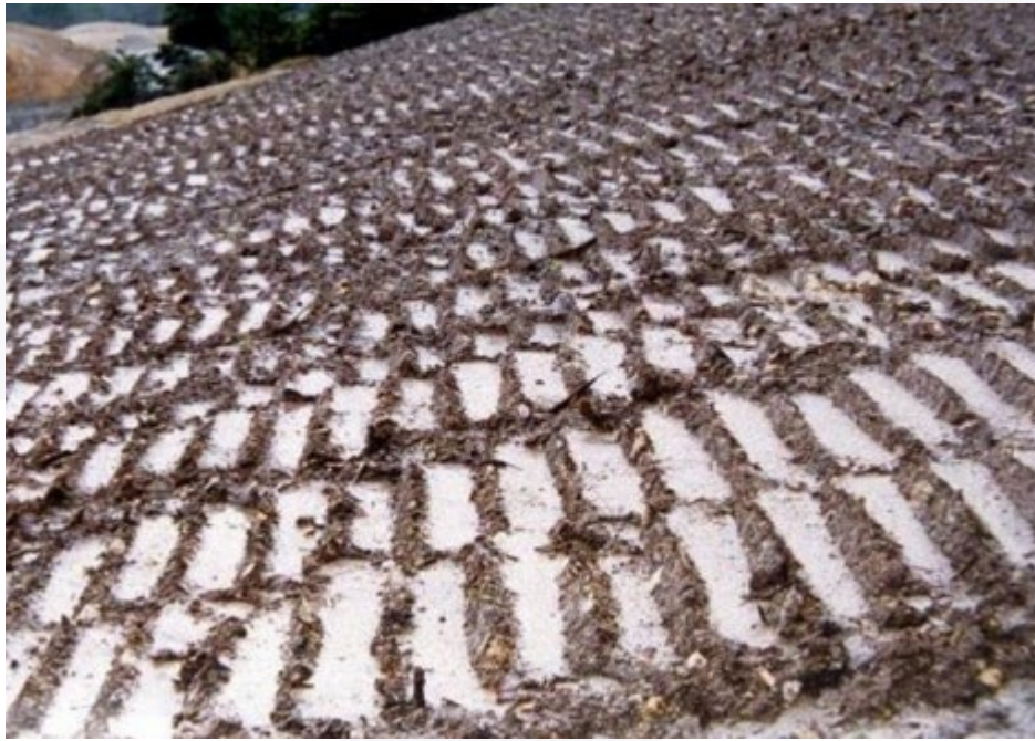
Figure 22: Surface Roughening of a Slope (Figure 39 from GD05)
