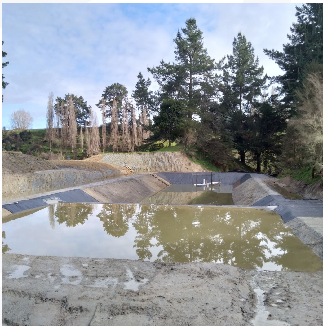
Figure 25: Example Sediment Retention Pond on a Hilly Site
