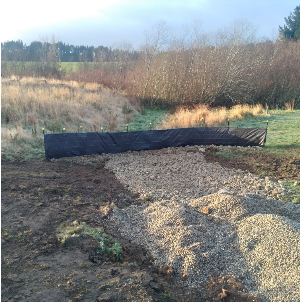
Figure 23: Example Silt Fence – Isolated Earthworks Area Adjacent to a Watercourse
