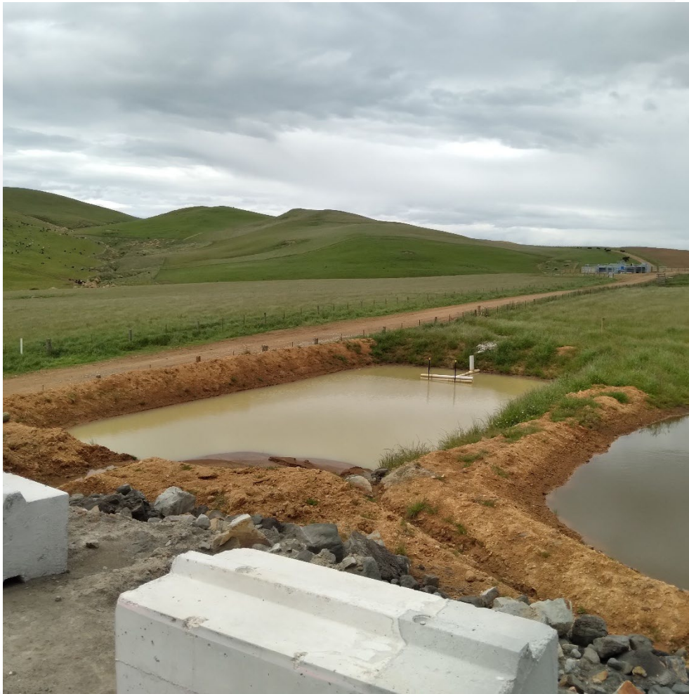
Figure 24: Example Decanting Earth Bund – Adjacent to a Construction Platform
