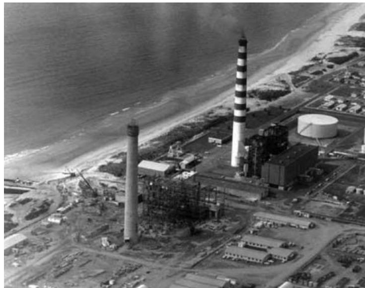
Marsden Point Power Station, Whangarei, Northland: 1976 Station B - Aerial View - during construction 6
