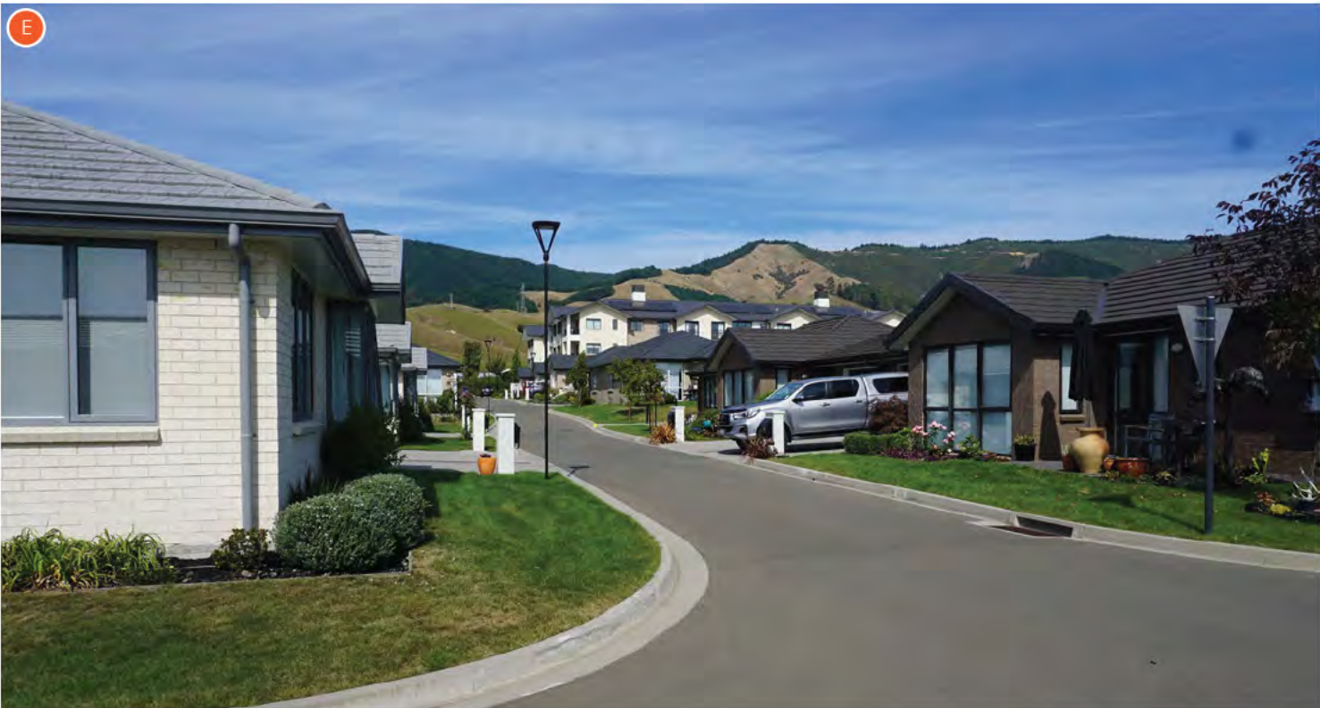
Summerset Richmond Ranges: This image was taken within Summerset Richmond Ranges, a sizeable retirement community which is currently under construction immediately to the east of the site. This development has recently, and is still in the process of re-defining Richmond's urban boundary, expanding it outwards.
