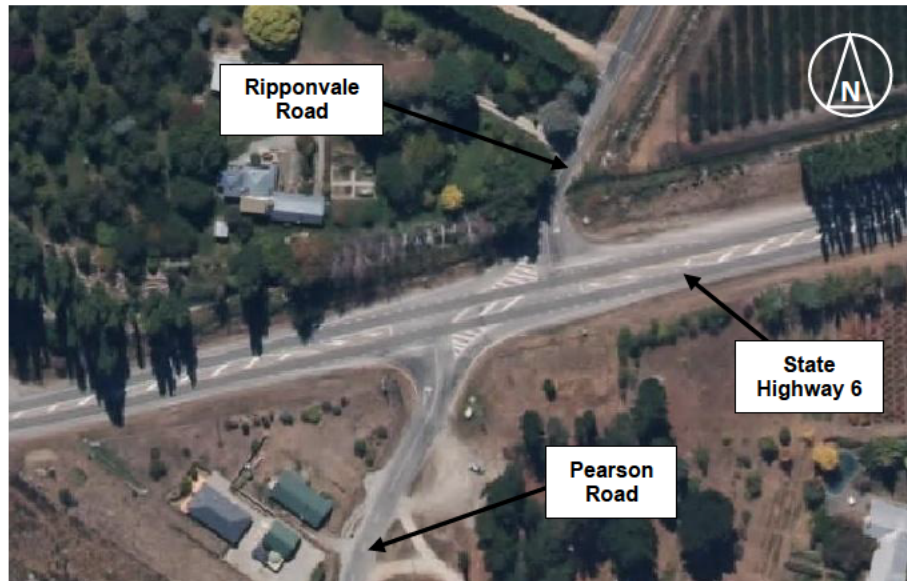
Photograph 7: Aerial View of the State Highway 6 / Ripponvale Road / Pearson Road Intersection
