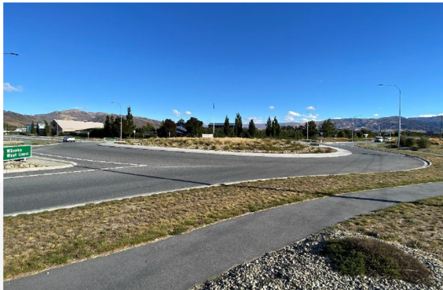
Photograph 6: State Highway 6 / State Highway 8B Roundabout Looking South
