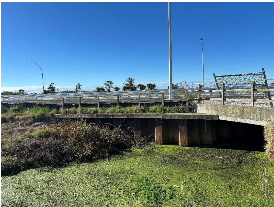
Figure 6: TEL Box Culvert (Source: Maven)
