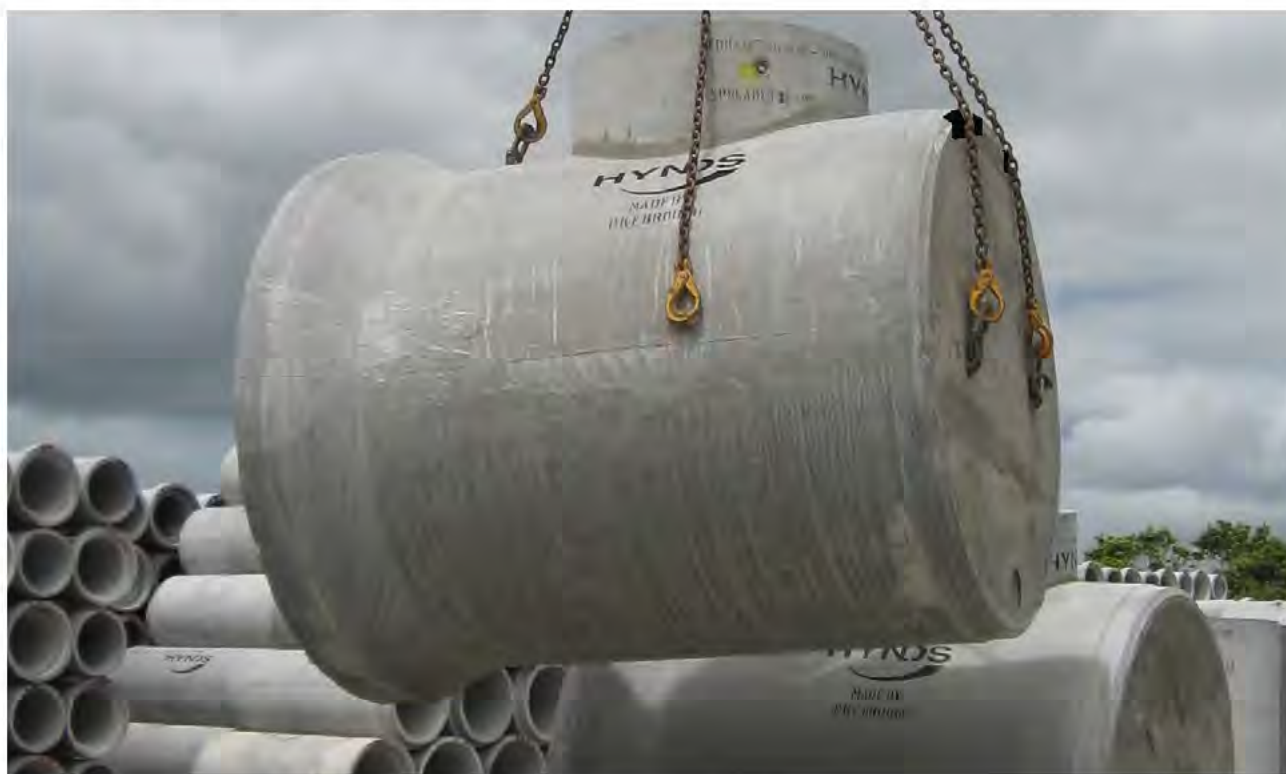
FIG. 6 Point lift of typical plugged end pipe
