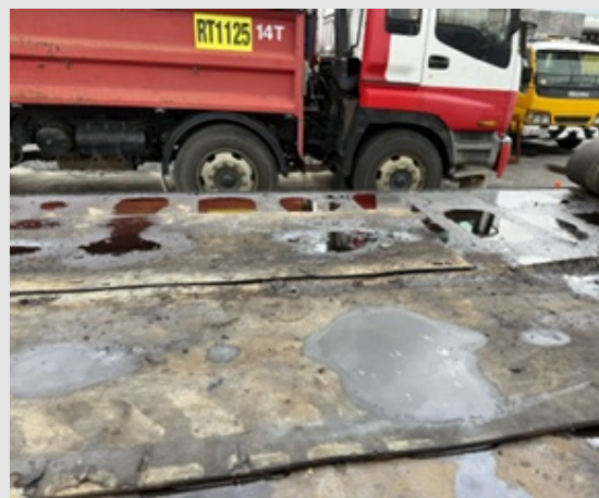
Bitumen truck storage
