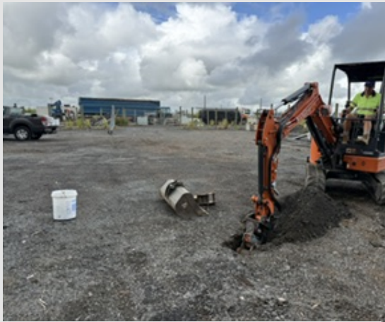
Test pitting in storage yards
