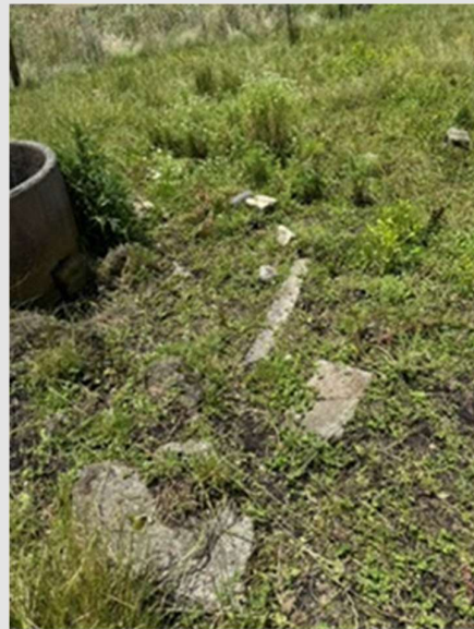
Suspected ACM debris in pasture in vicinity to toe of Latham's Mountain
