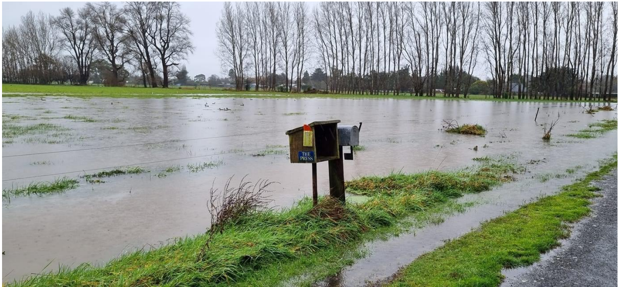
Flooding evidence Pictures taken July 2024 of the proposed subdivision site
