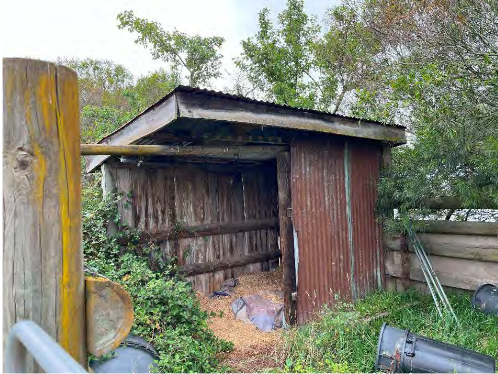
PLATE 7: North-eastern aspect of Shed 6.
