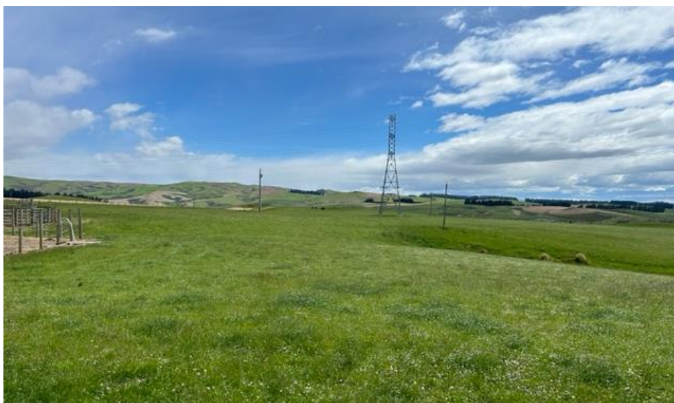
Figure 10. Tower 196 on HWB-ROX-A National Grid line viewed from Eldorado Track. The wind farm line will be connected directly to conductors on the pylon, requiring four adjacent poles, but avoiding a switch yard. The connection will be anchored by the farm stockyards on the left of the photo. The
