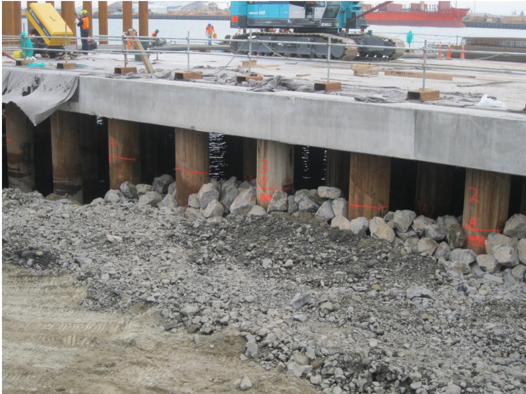
Figure 64: Rock armouring of batter slope viewed from behind the wharf.
