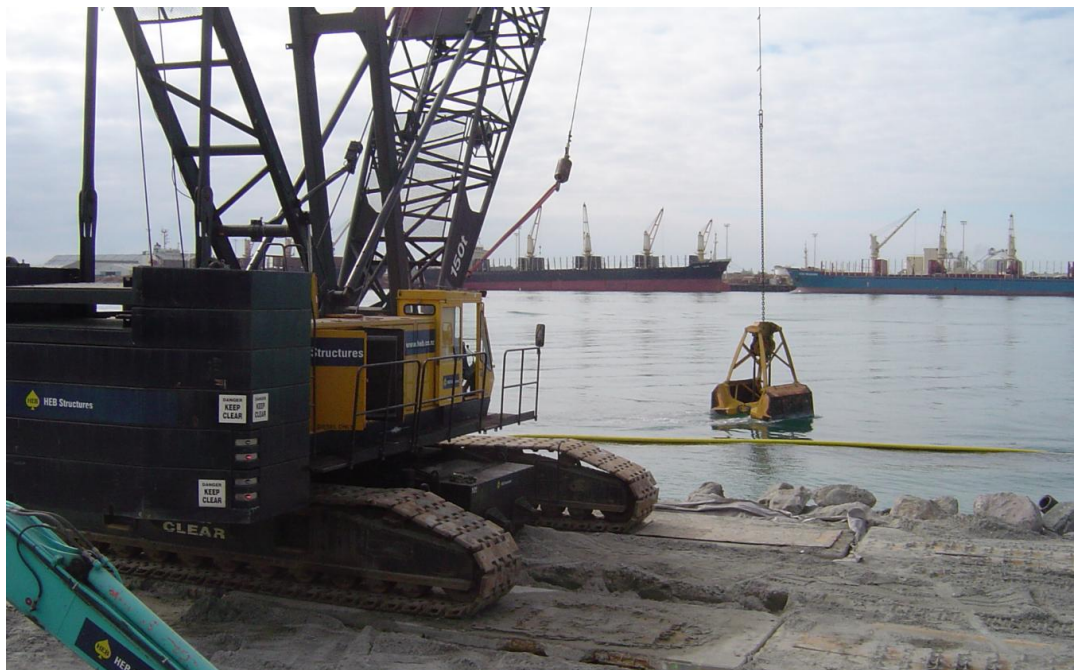
Figure 62: Excavation of batter slope by crane with grab.
