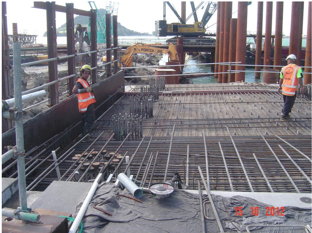
Figure 72: Deck formwork suspended off piles with reinforcing steel being placed.
