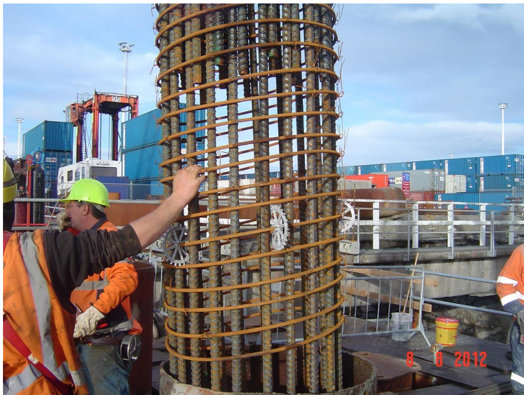
Figure 71: Reinforcing cage for steel pile.
