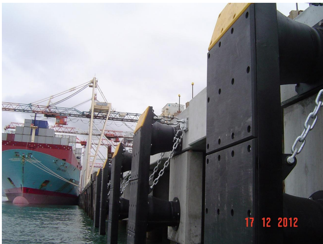
Figure 74: Fendering on the 2013 Sulphur Point extension.
