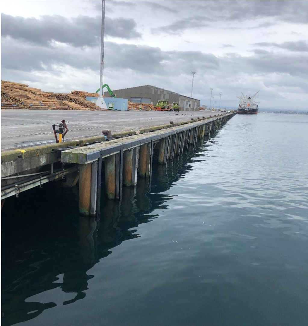
Figure 73: Fendering on the Mount Maunganui Wharves.
