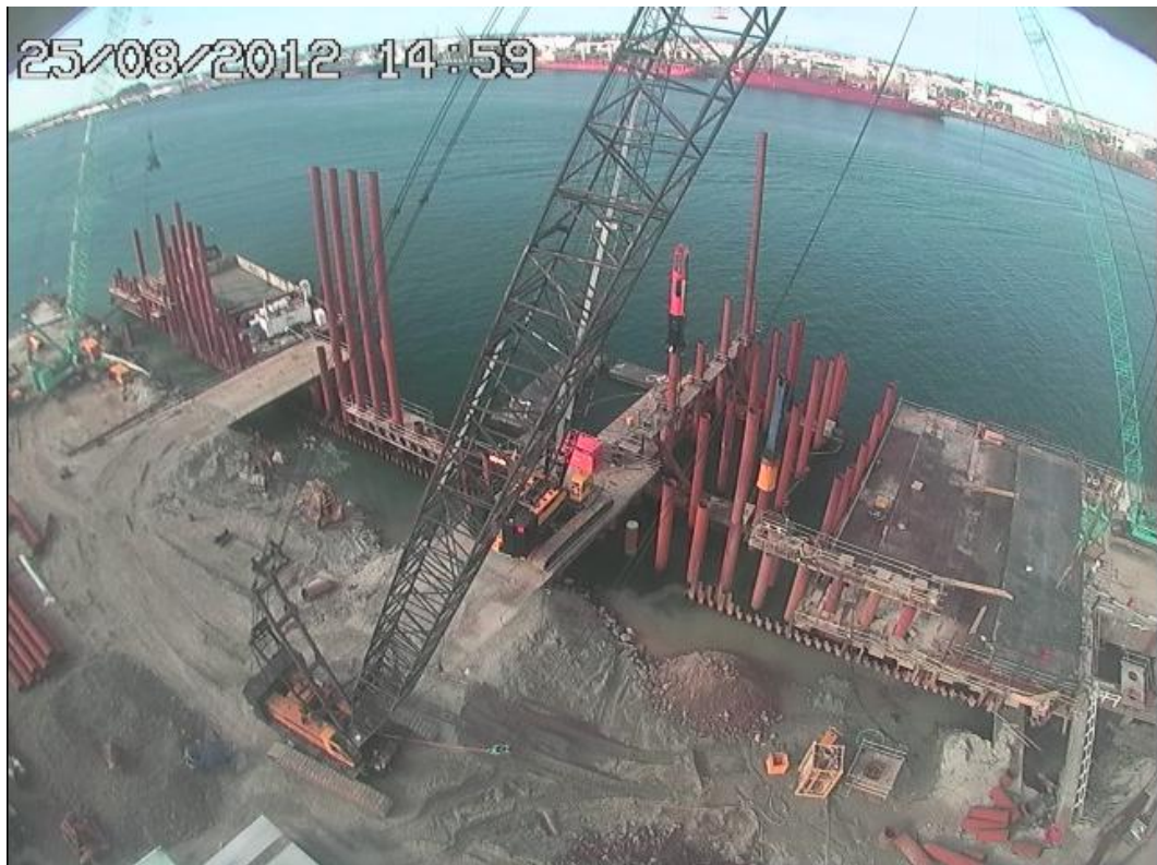
Figure 70: Pile driving operations at Sulphur Point in 2012.
