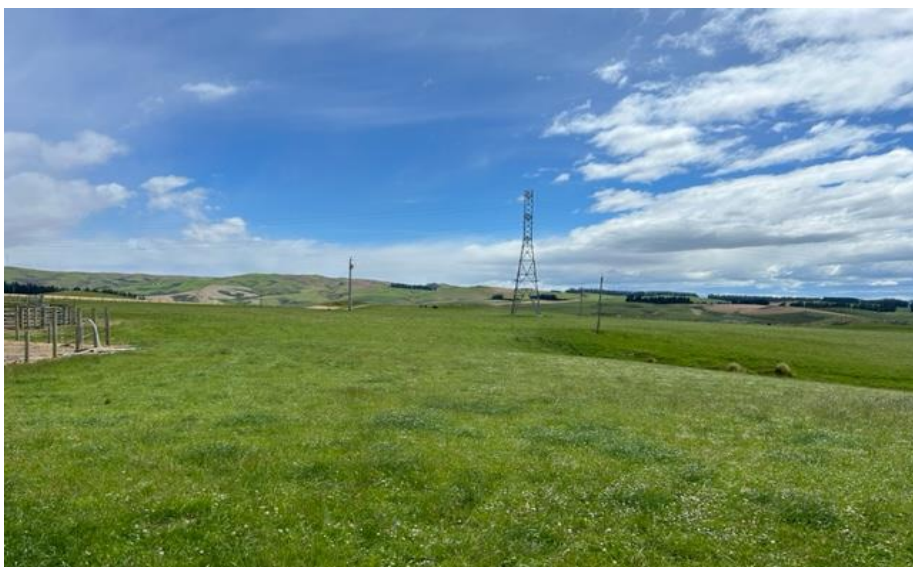
Figure 11: Tower 196 on HWB-ROX-A National Grid line viewed from Eldorado Track. The wind farm line will be connected directly to conductions on the pylon, requiring four adjacent poles, but avoiding a switch yard.
